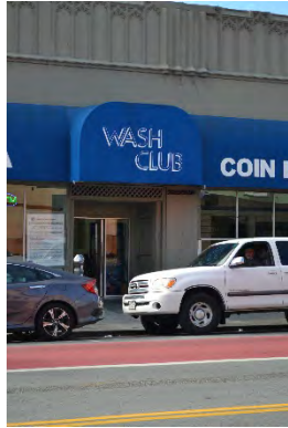
Figure 4. Glazed door and glazed sidelite, east (primary) façade, facing west
