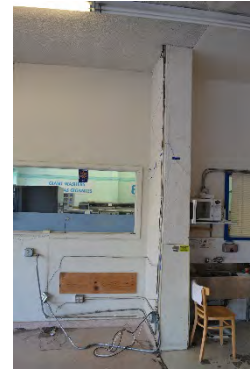
Figure 12. Two windows within the partition wall that separates laundry from vacant commercial space, facing south
