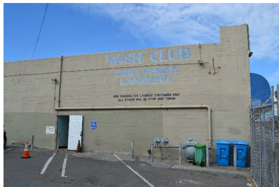
Figure 6. Entrance at the South façade, facing north
