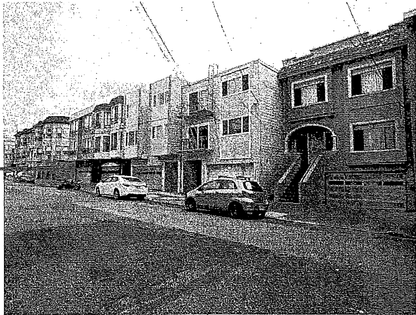
Same side of 27 th Avenue as 218 27 th Avenue, looking left. Arrow points to 218 27 th Avenue.
