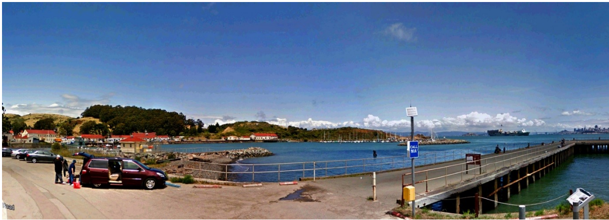
Figure 13 View of Fort Baker
