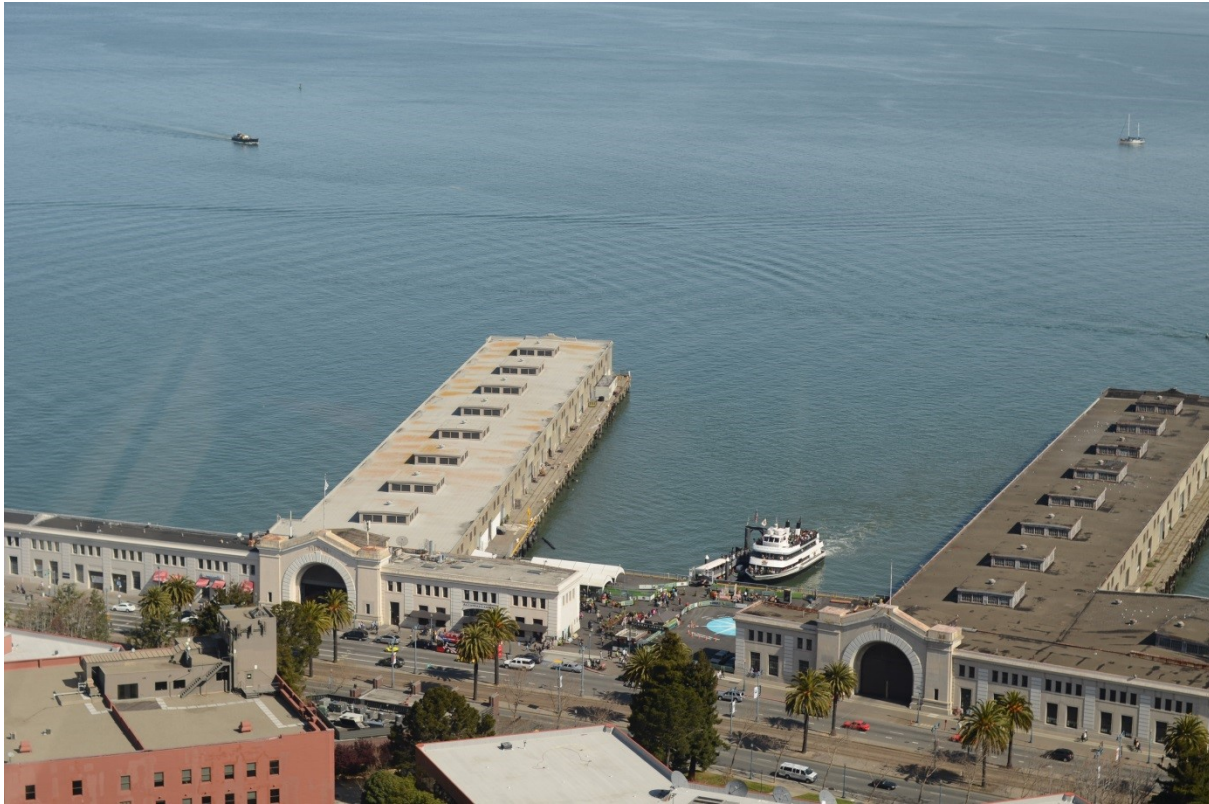
Figure 11 Existing View of Pier 31½ from Coit Tower
