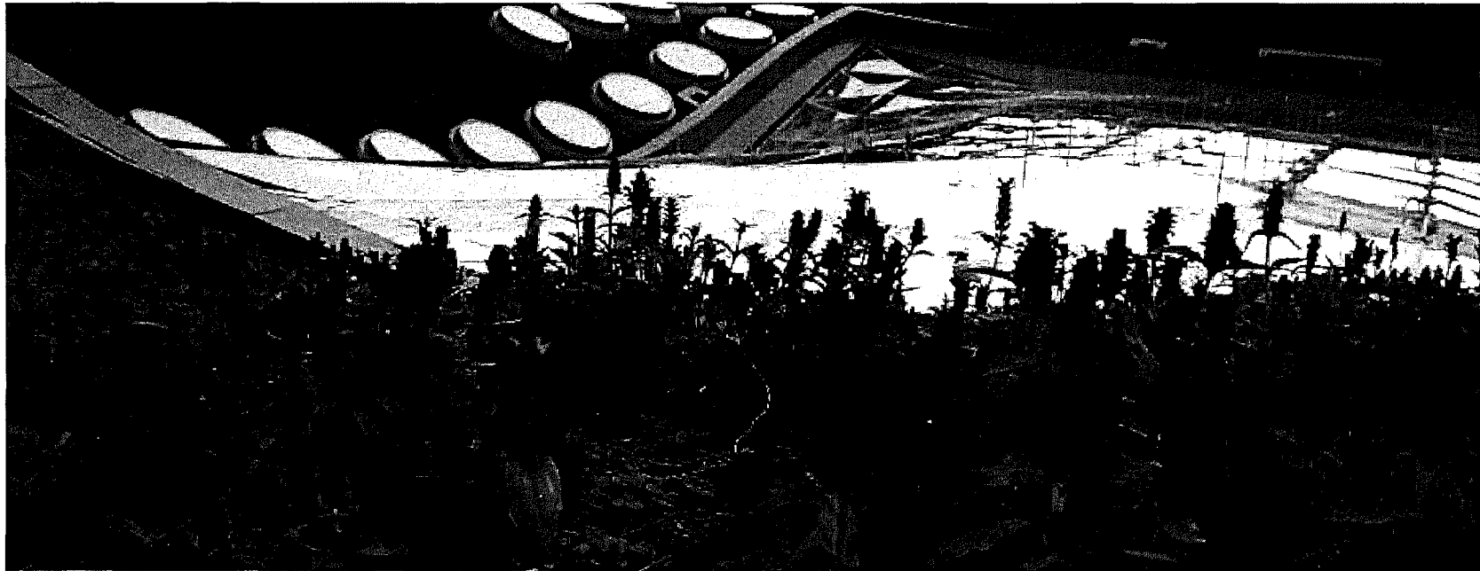
The Academy of Sciences in Golden Gate Park is targeting LEED Platinum certification and includes a 2.5 acre vegetated roof. Photo: Rana Creek - Living Architecture
