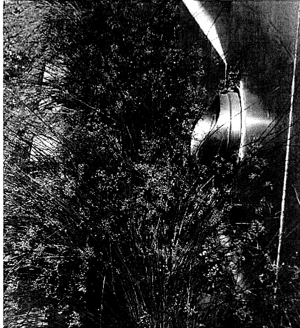
An interior roof drain discharges to a vegetated swale in Emeryville, CA. This properly designed and permitted stormwater facility is an example of an “approved alternate location” for stormwater discharge.
