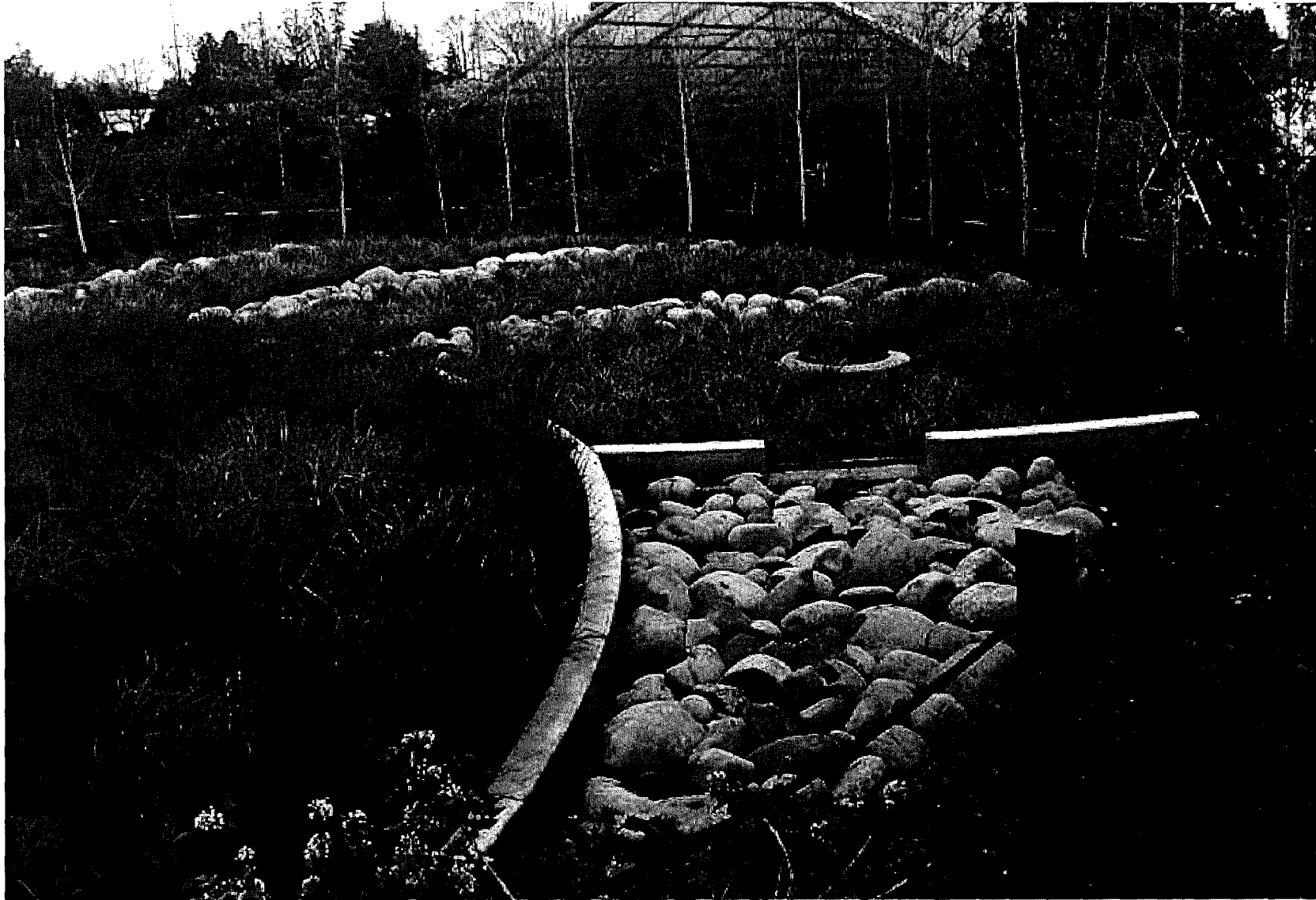
A rain garden at Glencoe Elementary in Portland, Oregon reduces stormwater flows to Portland's collection system.
