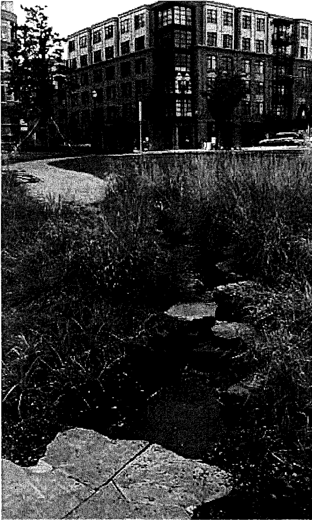
LID measures like the stormwater wetland in Portland's Tanner Springs Park treat polluted street runoff, thereby minimizing negative impacts to water quality.
