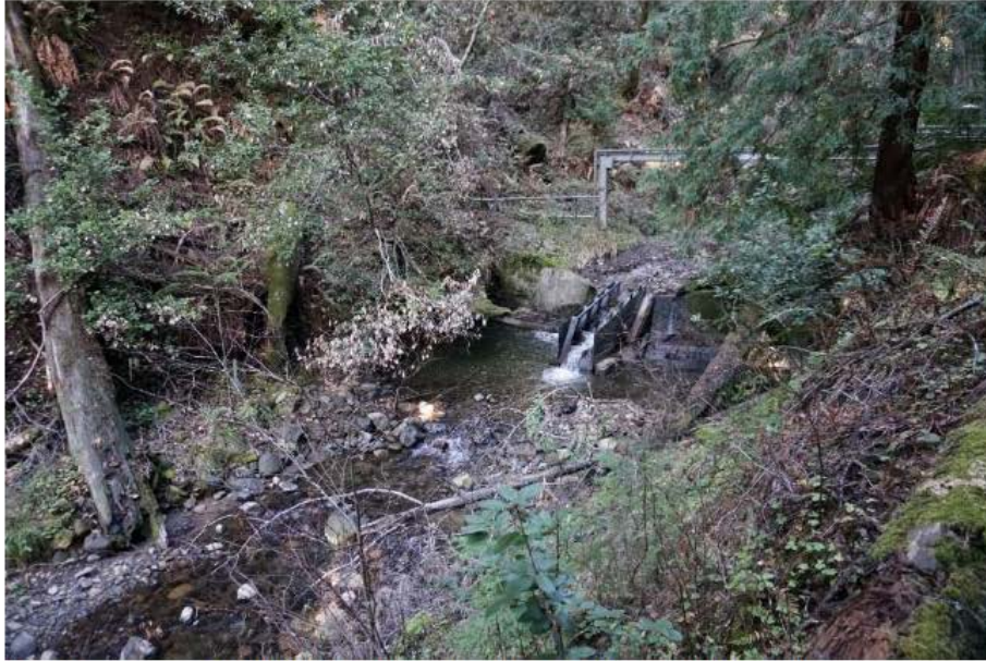
Photo 1: Dam and Denil ladder facing upstream, February 2020
