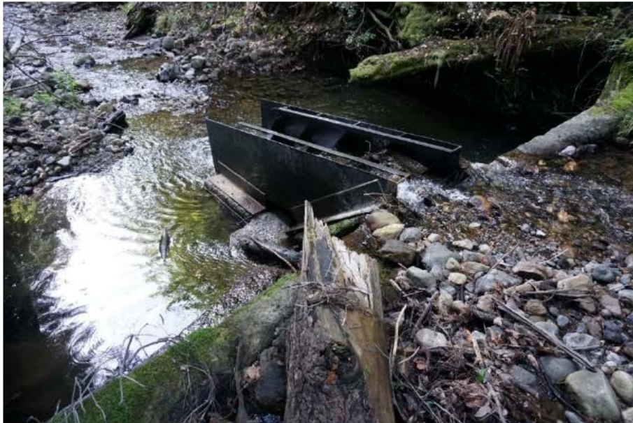
Photo 2: Dam and Denil ladder facing downstream, February 2020
