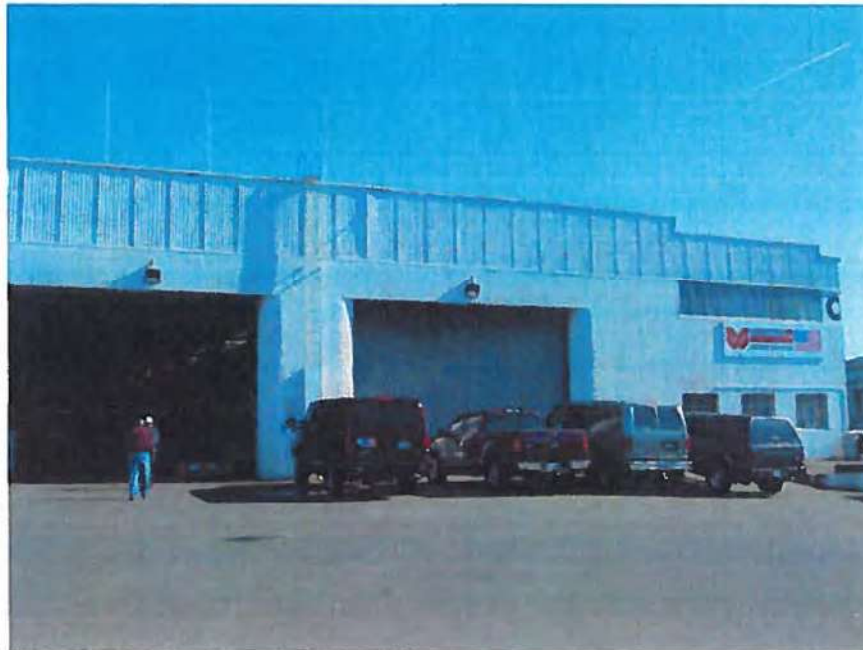
Photo 2. Partial west elevation
