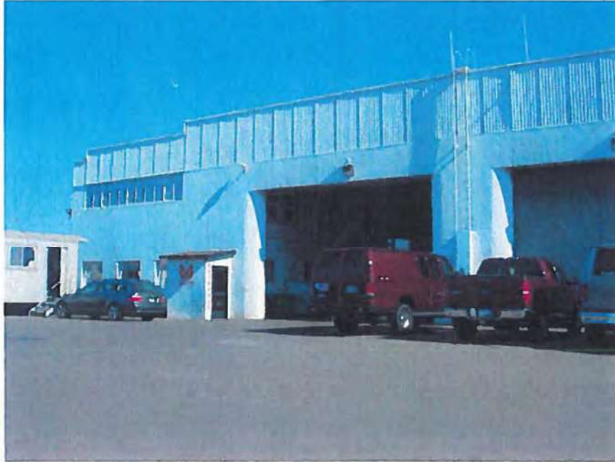
Photo 1. Partial west elevation
