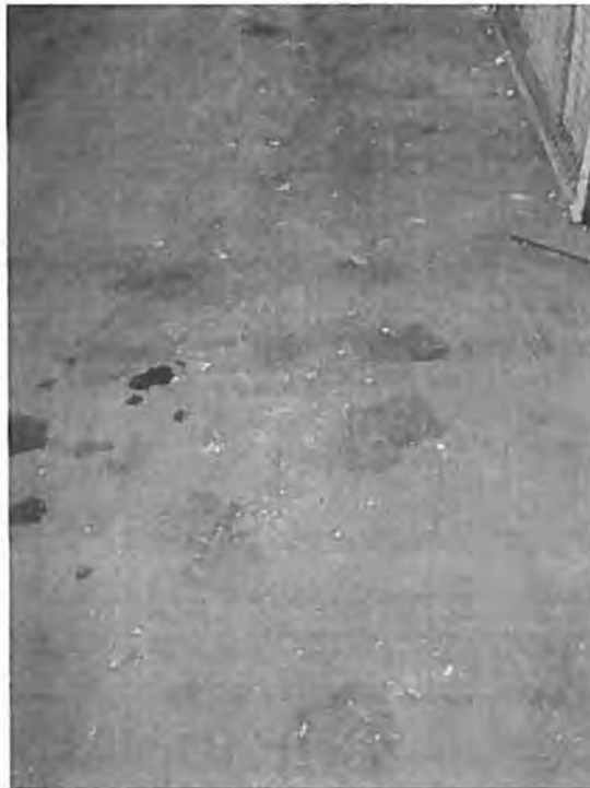
Photo 4. Peeled paint from roof wood trusses
