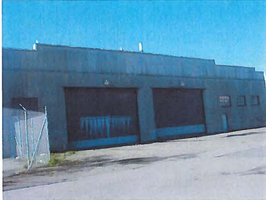
Photo 7. Partial east elevation
