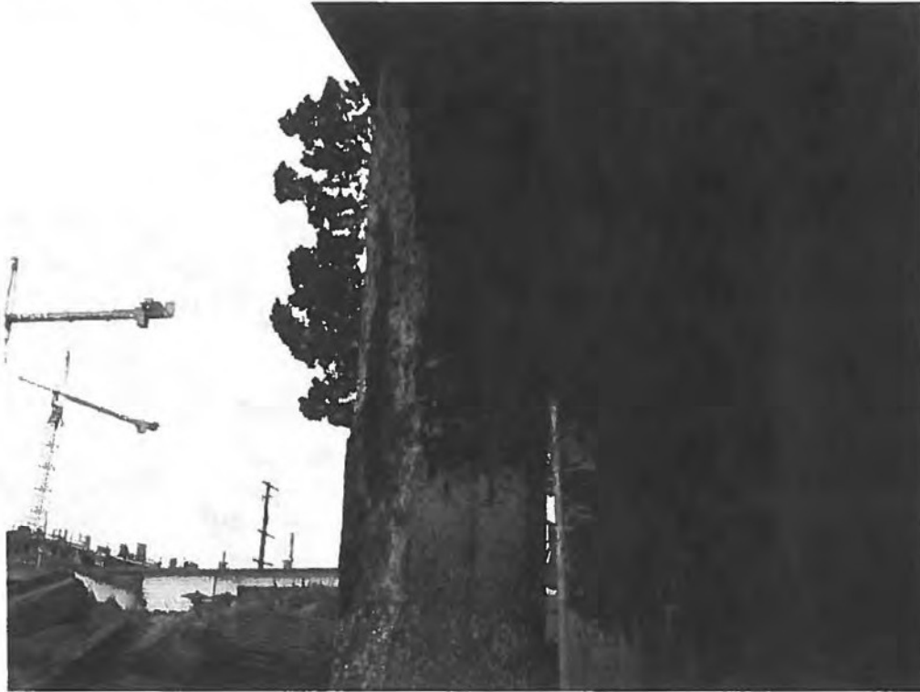
Figure 3: Pile, spalling
