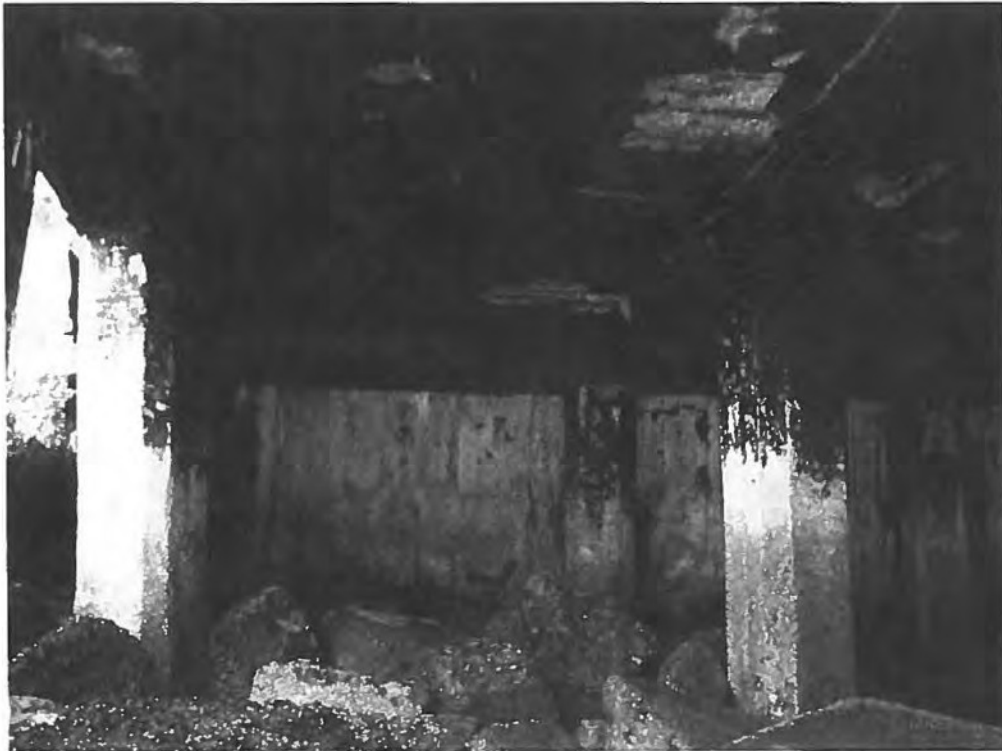
Figure 7: Piles, rip-rap, seawall
