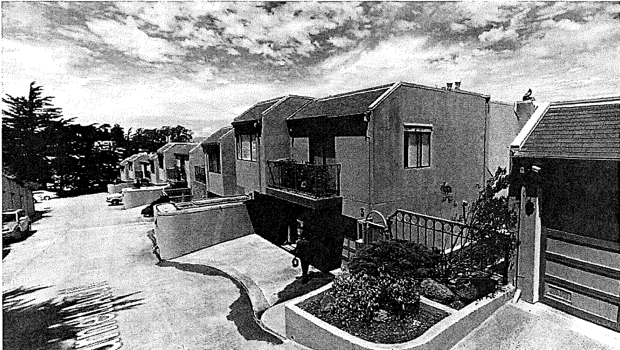
1 – 20 Burnett Avenue North is a condominium complex with one story over a garage at the street and contains four floors to the rear.
