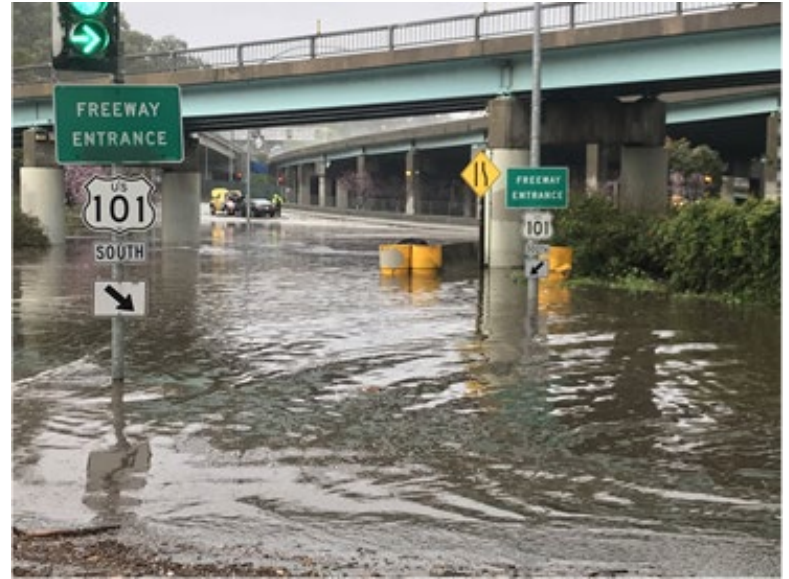
Flooding in Lower Alemany Area
