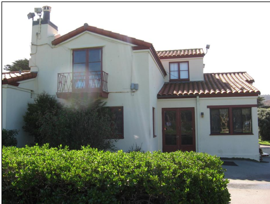
Photograph 9: North side of clubhouse, camera facing south, 3/4/2010
