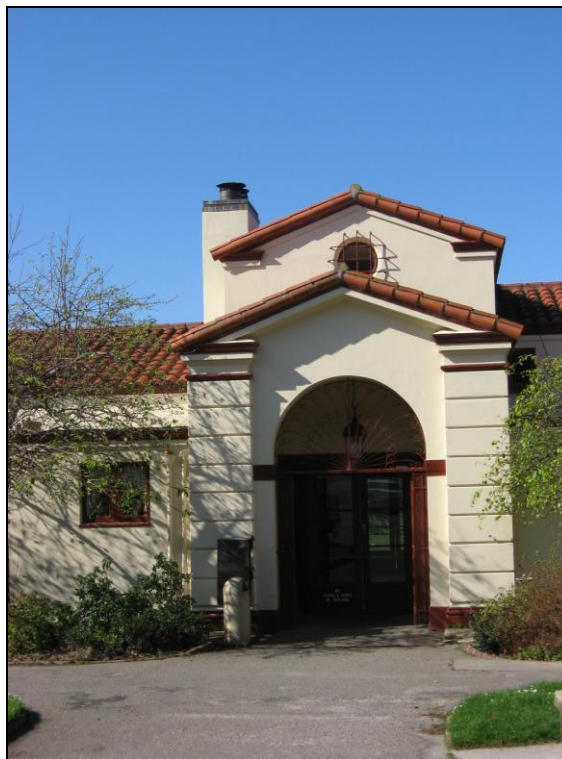
Photograph 7: East entrance to clubhouse, camera facing west, 3/4/2010
