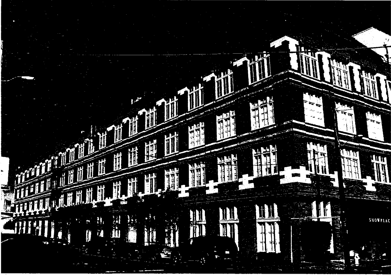
West facade (l), south facade (r)
