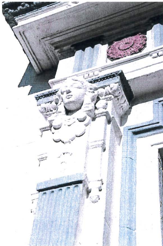
Pilaster detail, 2014, Christopher VerPlanck
