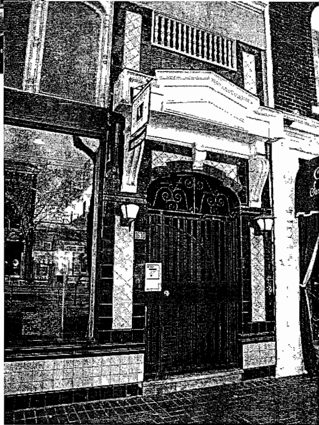
Figure 22 - 1670 Market Street entry detail
