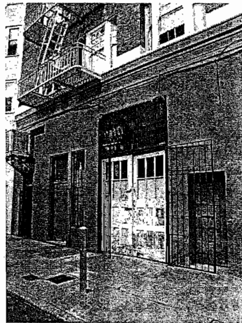
Figure 12 - 1649 Market Street, Stevenson St. detail
