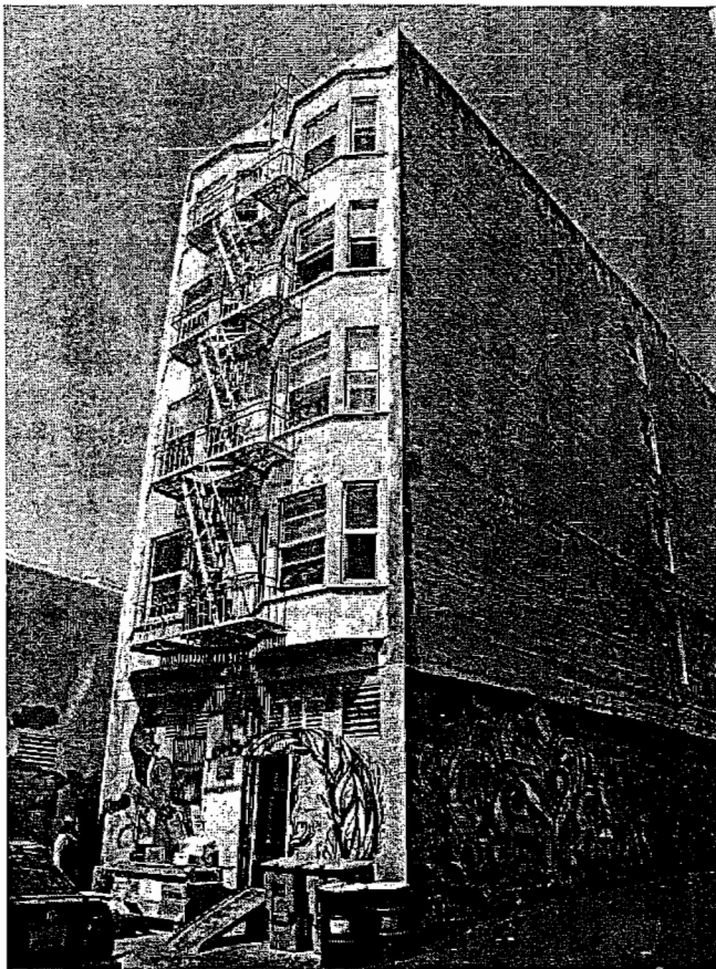
Figure 29 - 1693 Market St., Stevenson St. elevation
