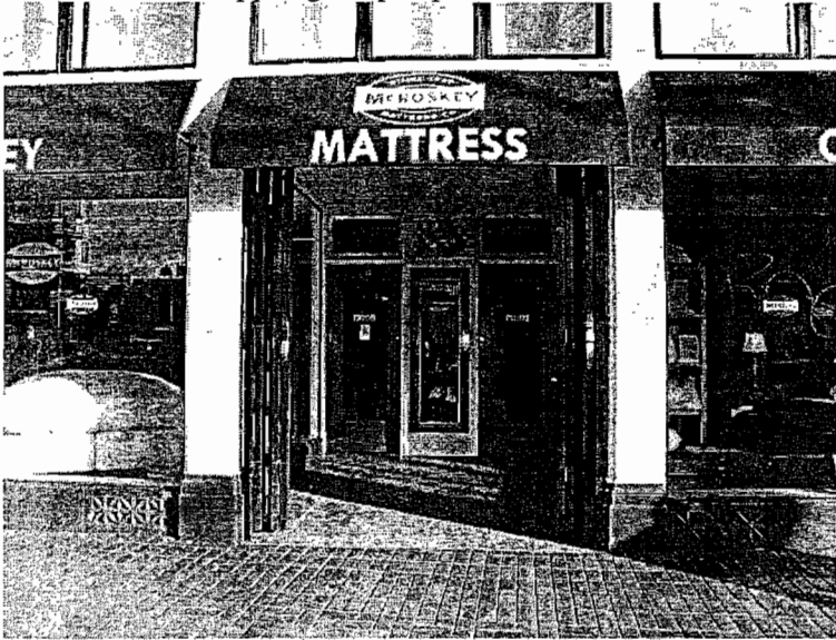
Figure 25 - 1687 Market St., entry detail
