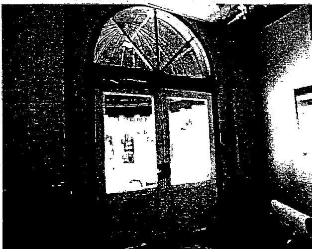
Interior of Montgomery Street entrance
