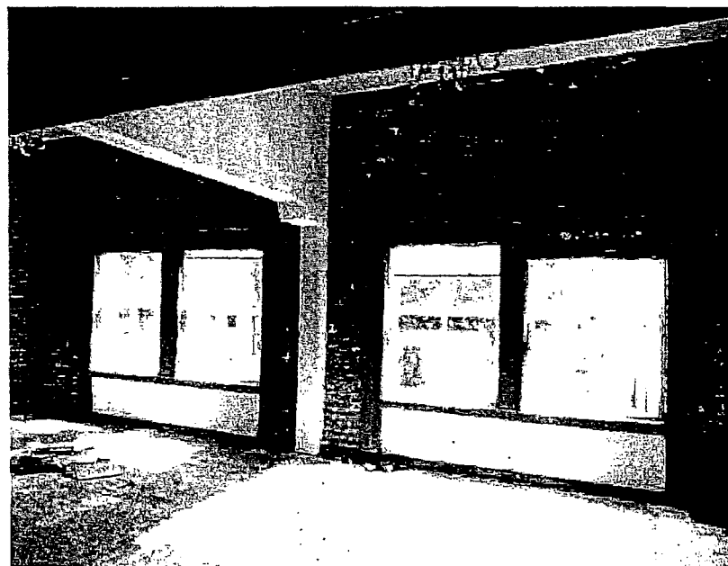
Interior of 2 nd Floor Montgomery Street windows
