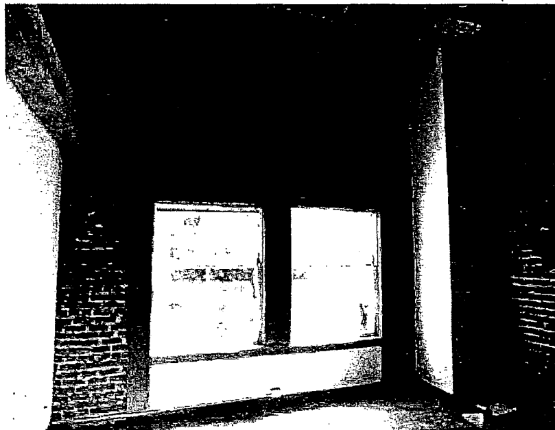
Interior of Montgomery Street 2 nd Floor windows
