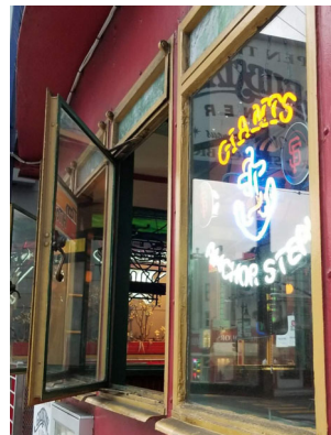
EXISTING GRUBSTAKE WINDOWS - TO BE REUSED
