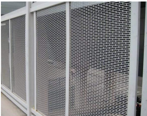
PERFORATED METAL PANEL / GUARDRAIL
