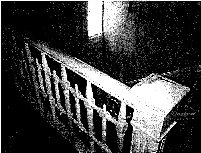
Additional Subject Photo
