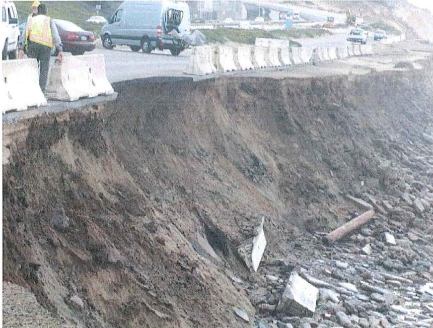
Figure 2. Eroding shoreline and rubble at South Ocean Beach, February 2016.
