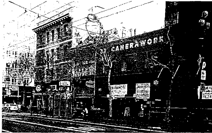
Figure 1. View east showing the Walker Building in its context on the south side of Market Street. [No. 15.54.33] January 2014.
