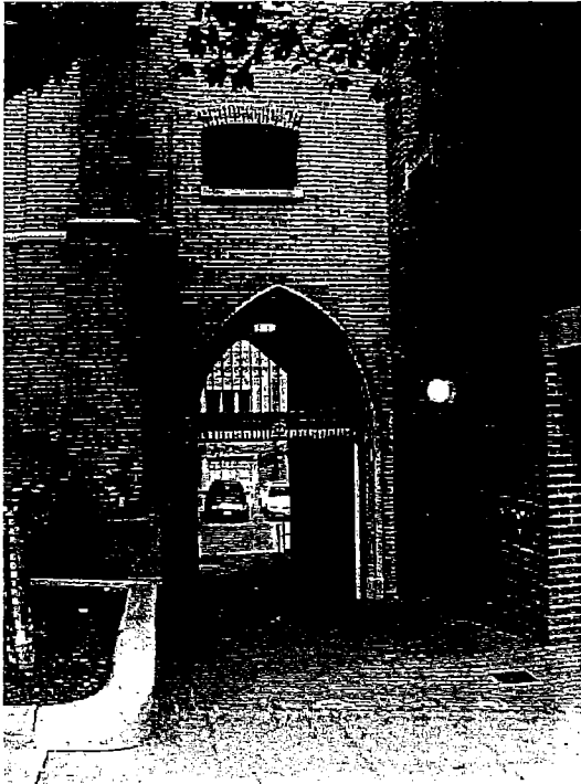
Entry to the parking lot below covered bridge which connects the rectory (right) to the sanctuary (left). (Page & Turnbull, March 2013)
