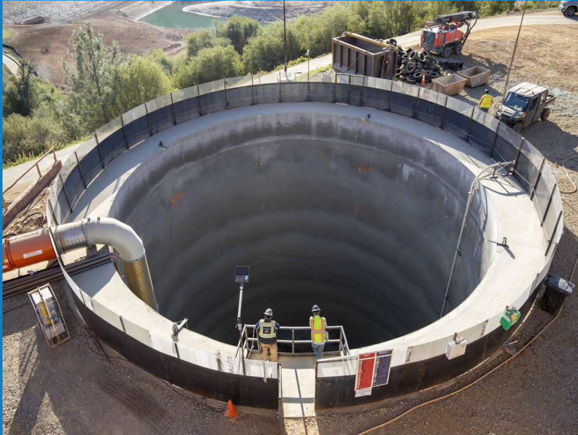
Flow Control Facility Shaft Under Construction
