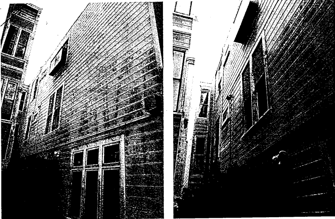
Figure 3: Views looking southeast at the north façade
