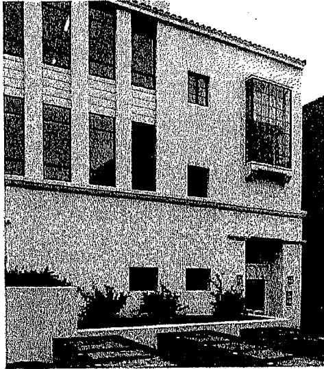
Figure 20 - Variety of windows on the south facade, all in good condition after the rehabilitation. Photo by Page & Turnbull
