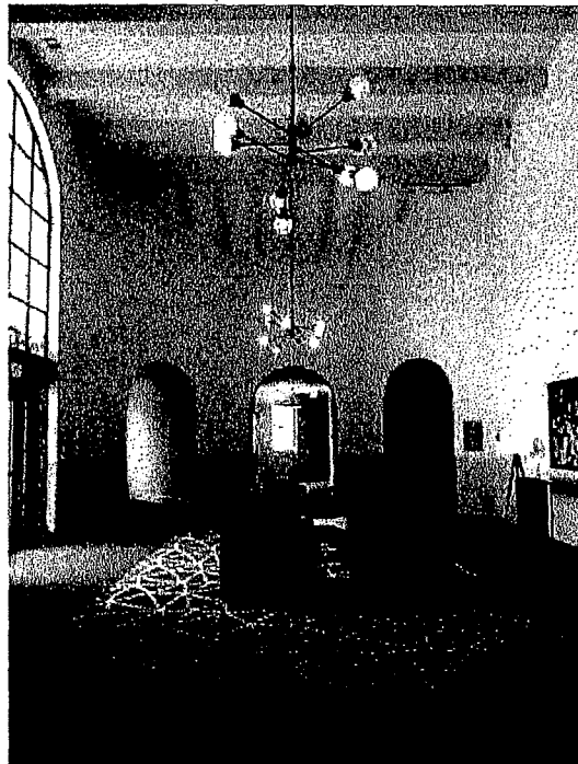
Figure 19. The main lobby interior carpeted and painted. Photo by Page & Turnbull, 2017
