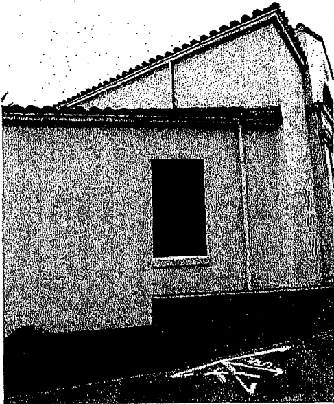
Figure 12 - The downspout from the upper roof sheds water onto this area of the lower roof, which bypasses the gutter and spills onto the ADA ramp into the Entry Pavilion. Photo by Page & Turnbull, 2017.
