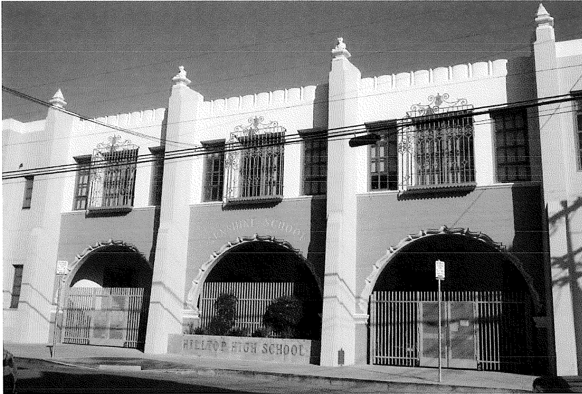
Figure 22. Central section of the west façade of the former Sunshine School; view toward northeast.
