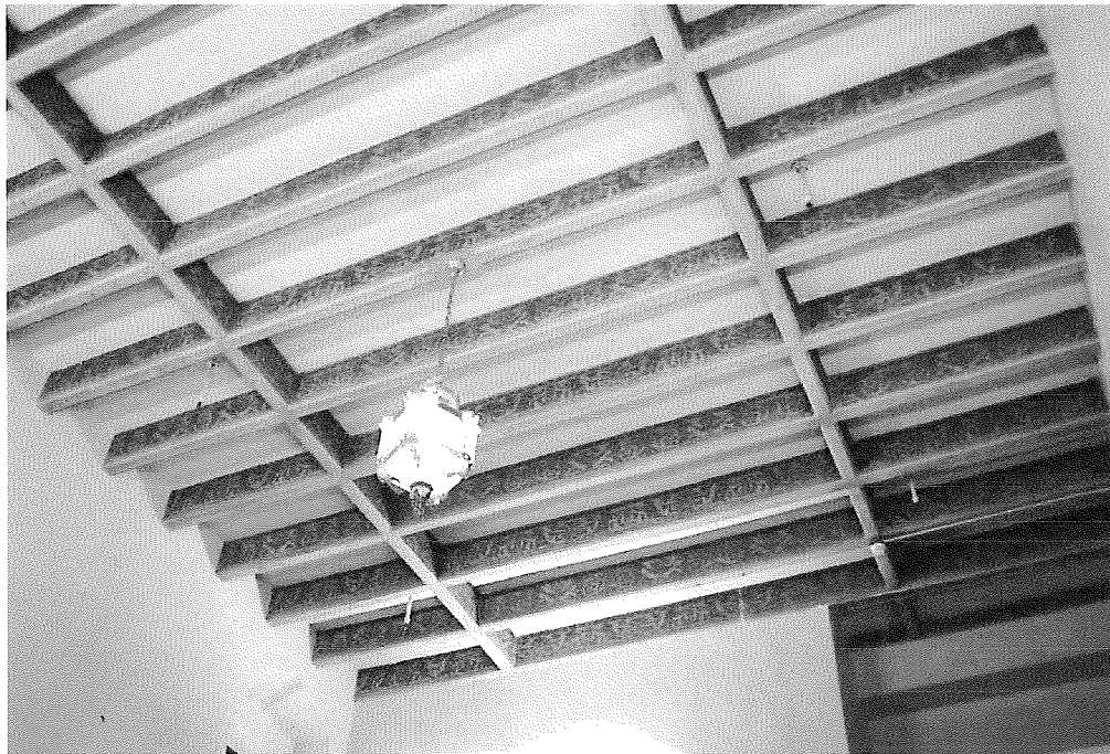
Figure 35. Ceiling of main lobby/stair; view toward north.
