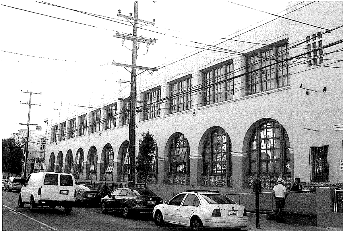
Figure 14. East façade of the Sunshine School (classroom wing); view toward southwest.
