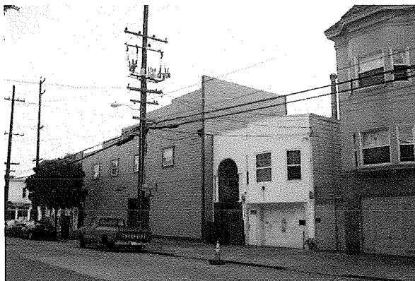
Figure 10. The south side of 25 th Street between Florida and Bryant Streets, north of the former Sunshine School, view toward southeast.
