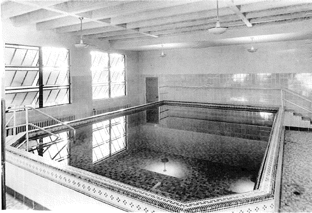
Figure 56. Therapeutic pool on first floor level of the Sunshine School, ca. 1937.
