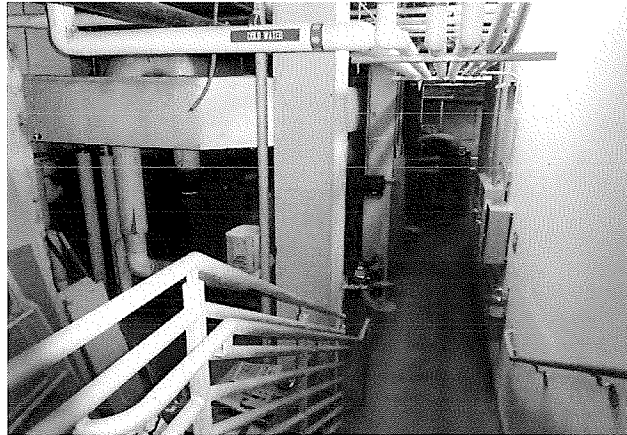
Figure 44. Basement of the former Sunshine School; view toward west.
