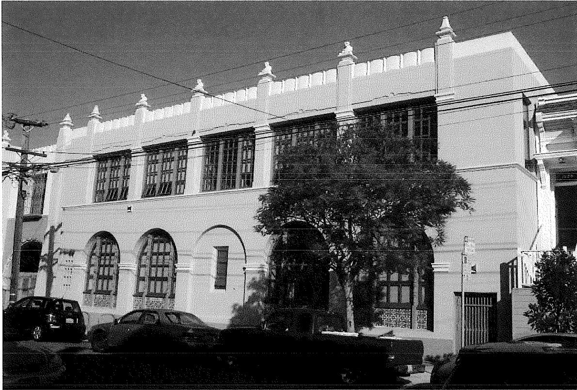
Figure 20. South part of the west façade of the former Sunshine School; view toward northeast.
