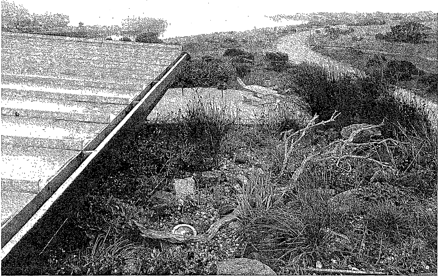
A vegetated roof and other LID features at the Eco-Center at Heron's Head Park help illustrate sustainable design practices to students in San Francisco's Bayview-Hunters Point neighborhood. Photo: Rosey Jencks
