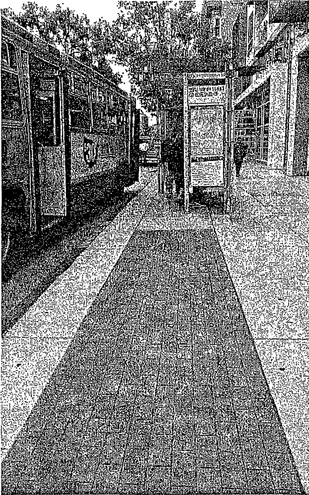
Permeable pavers along Van Ness Ave in San Francisco, CA. Photo: Krystal Zamora
