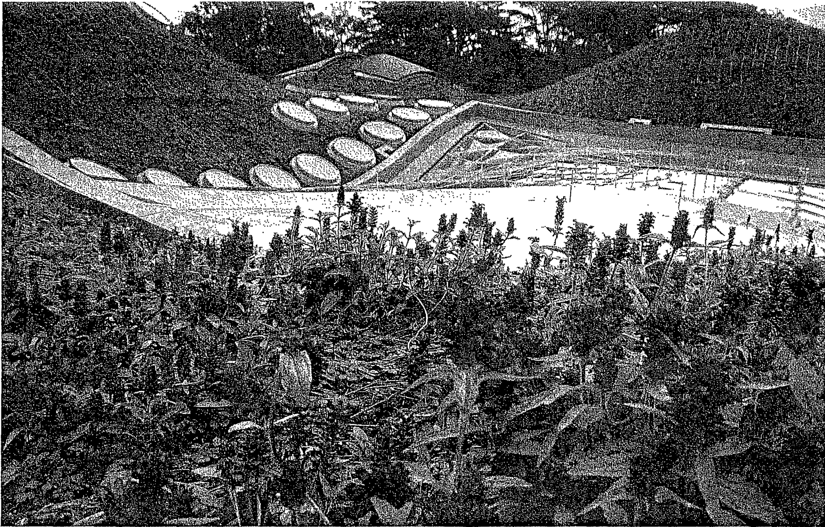
The Academy of Sciences in Golden Gate Park is a LEED Platinum building and includes a 2.5-acre vegetated roof. Photo: Rana Creek – Living Architecture
