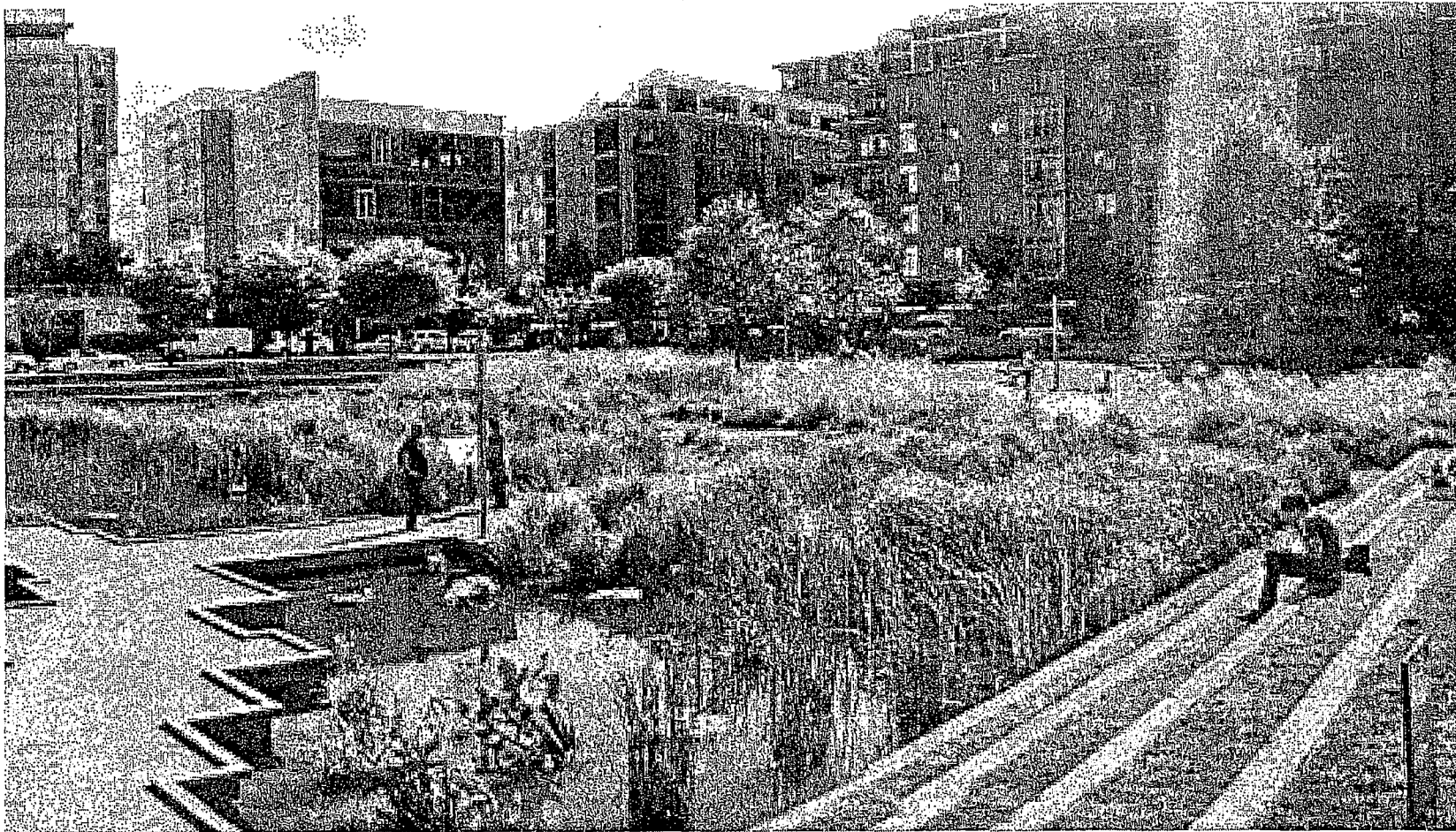
Green infrastructure BMPs such as the stormwater wetland in Portland's Tanner Springs Park treat polluted sidewalk runoff, thereby minimizing negative impacts on water quality. Photo: Rosey Jencks
