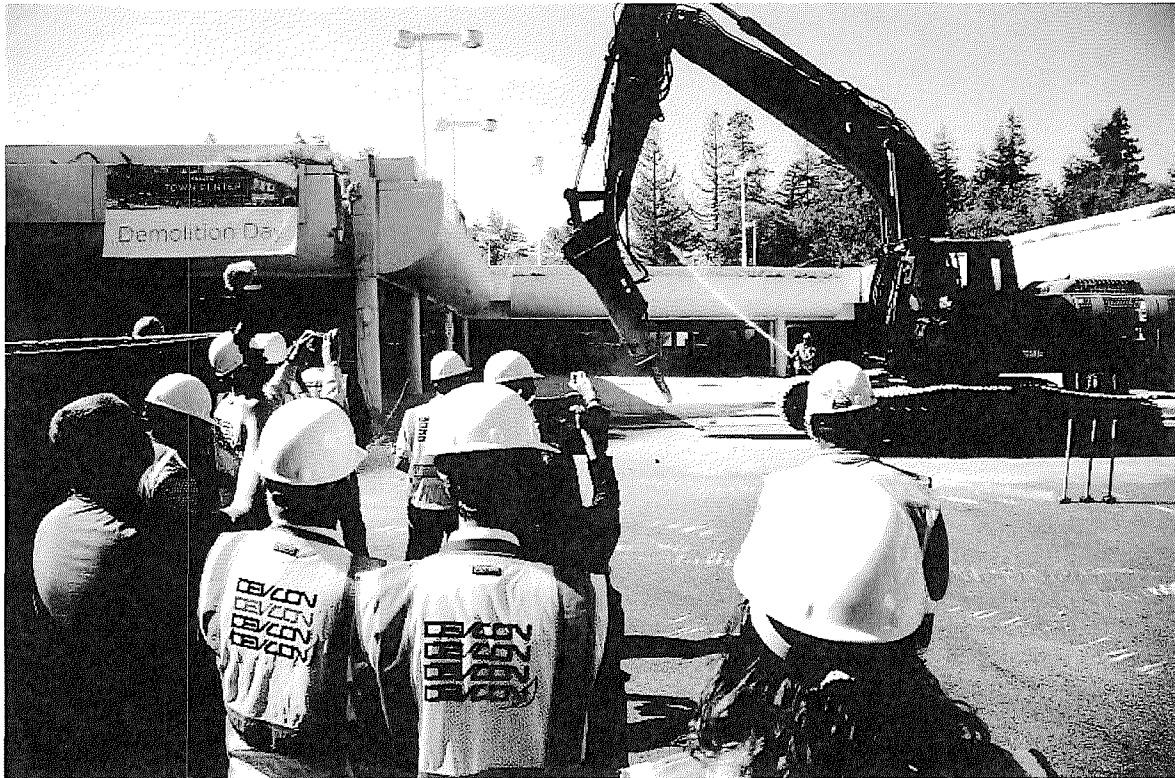
Demolition of a parking structure at the Vallco Shopping Mall began on Thursday, Oct.11, 2018, after an hour-long press conference celebrating the milestone in Cupertino, Calif. (Karl Mondon/Bay Area News Group)
