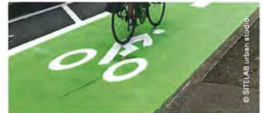
Standard asphalt with green surfacing
