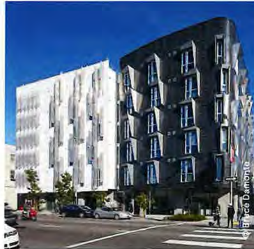
Change in roofline, articulation, and material
