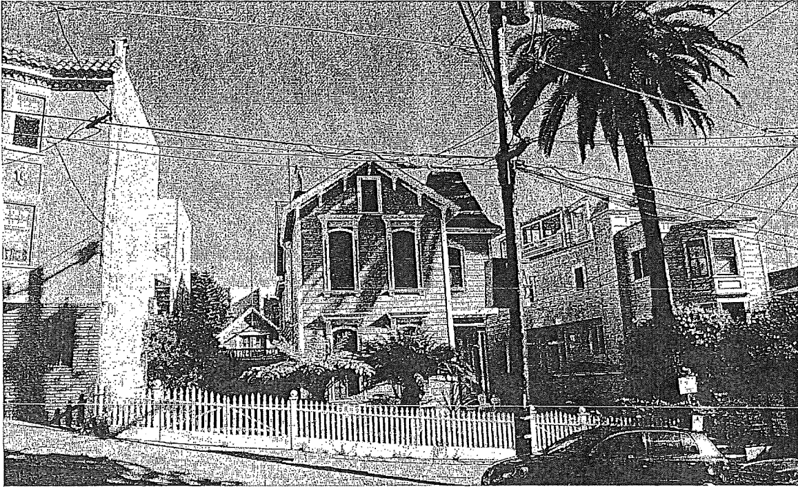
Figure 20. Overall view of 22 Beaver Street; view toward north.
