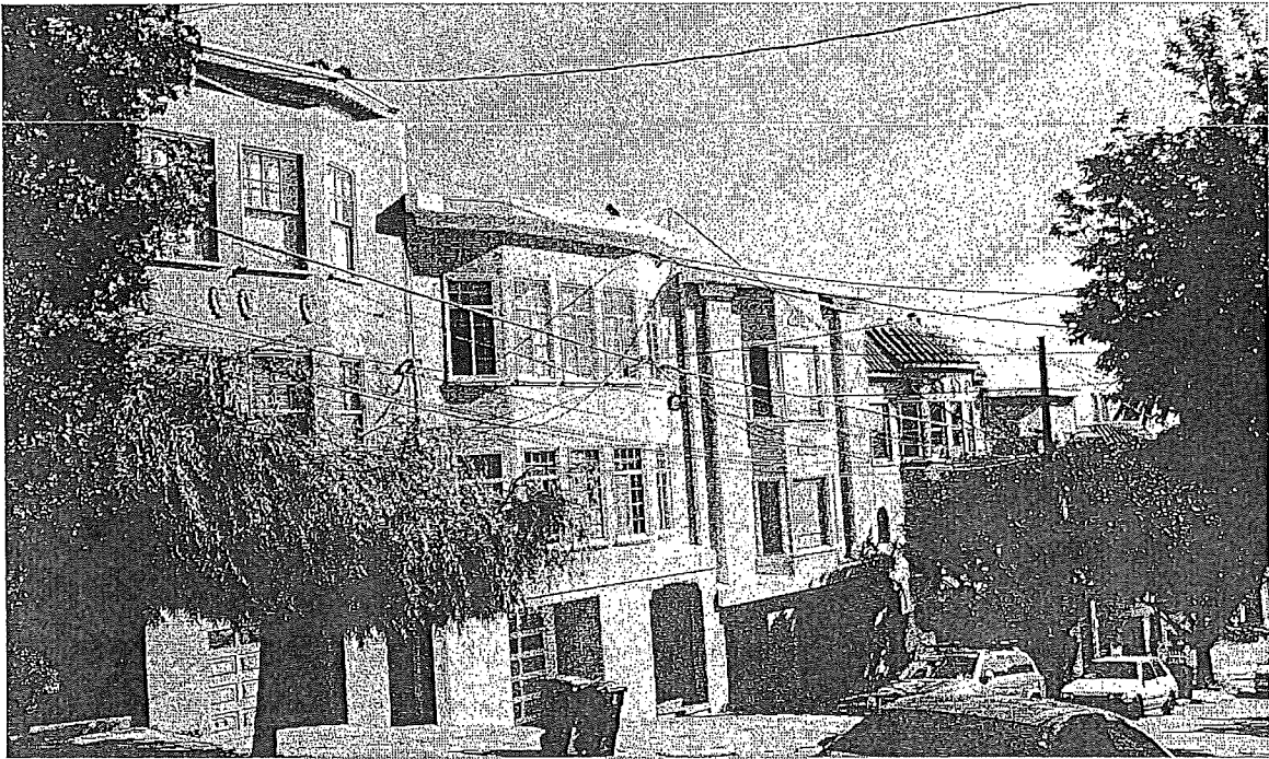
Figure 13. Row of Mediterranean-style flats at 46-48 to 68-70 Beaver Street; view toward northeast.
