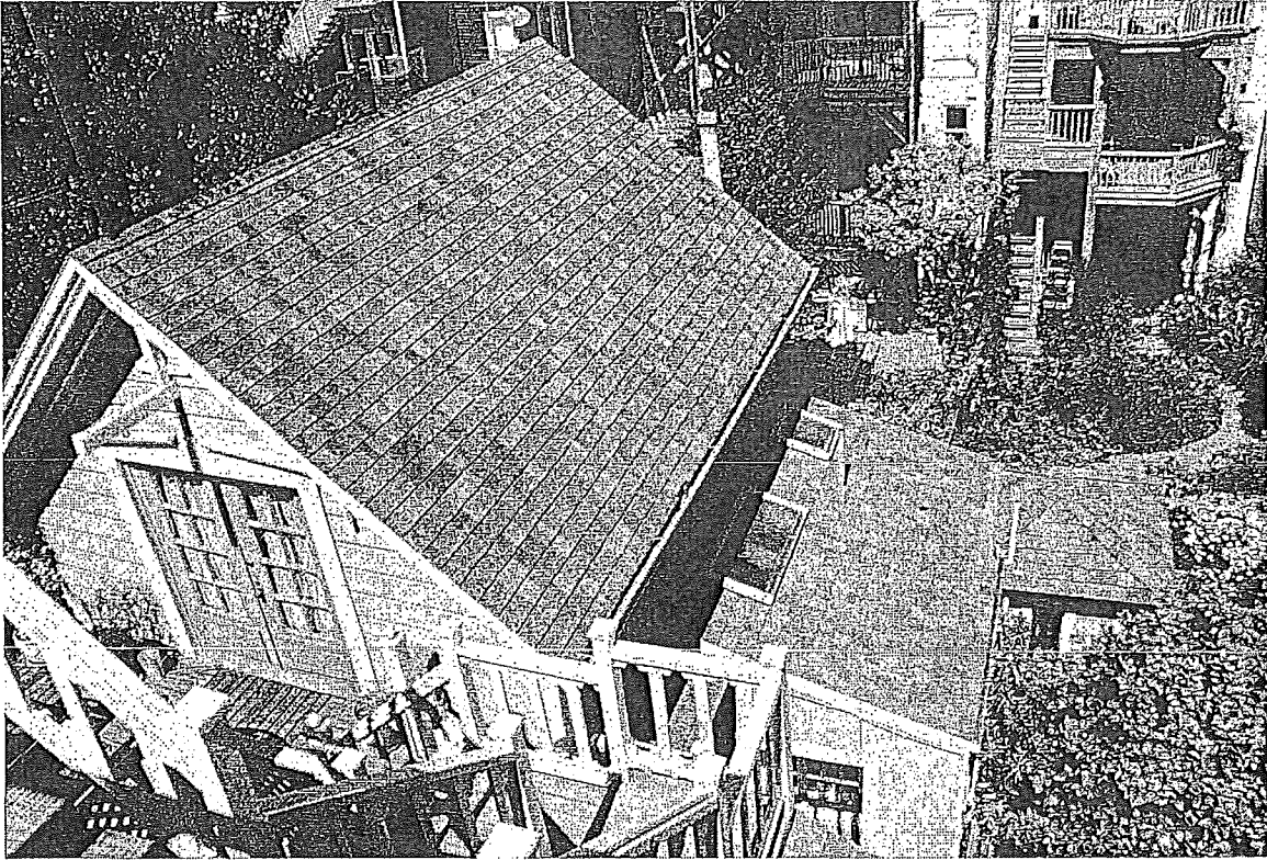
Figure 53. Garage/carrriage house; view from attic of main house; view toward northwest.
