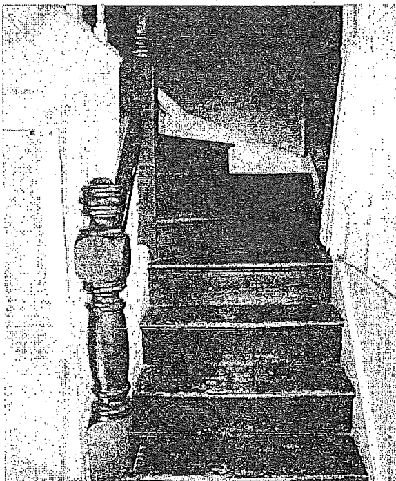
Figure 50. Attic stair; view toward north.
