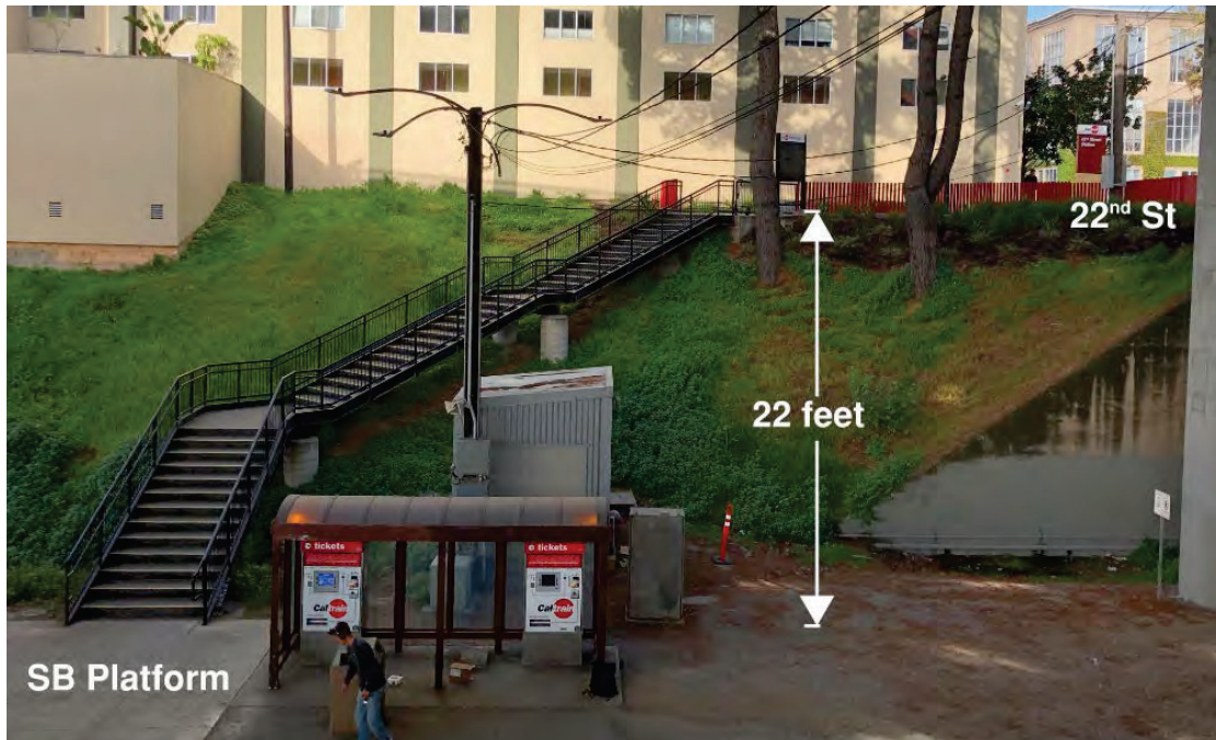
Southbound Platform Staircase
