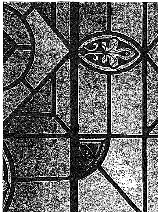
Figure 76. Detail, stained glass window. (Page & Turnbull, 05/25/2018)
