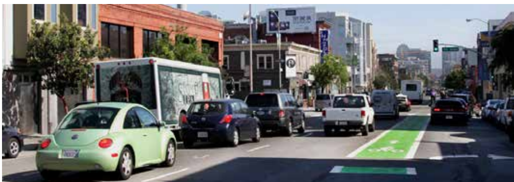
Progress photo of Folsom Street/Howard Street Streetscape Project
