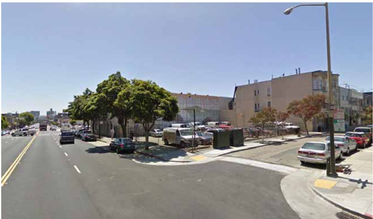
FIGURE 2.6 260 5th Street (2009, Before Construction)
