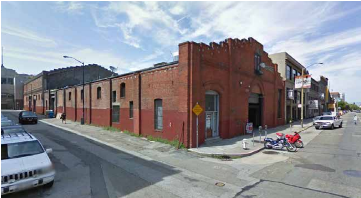
166–178 Townsend St (2009, Before Construction)
