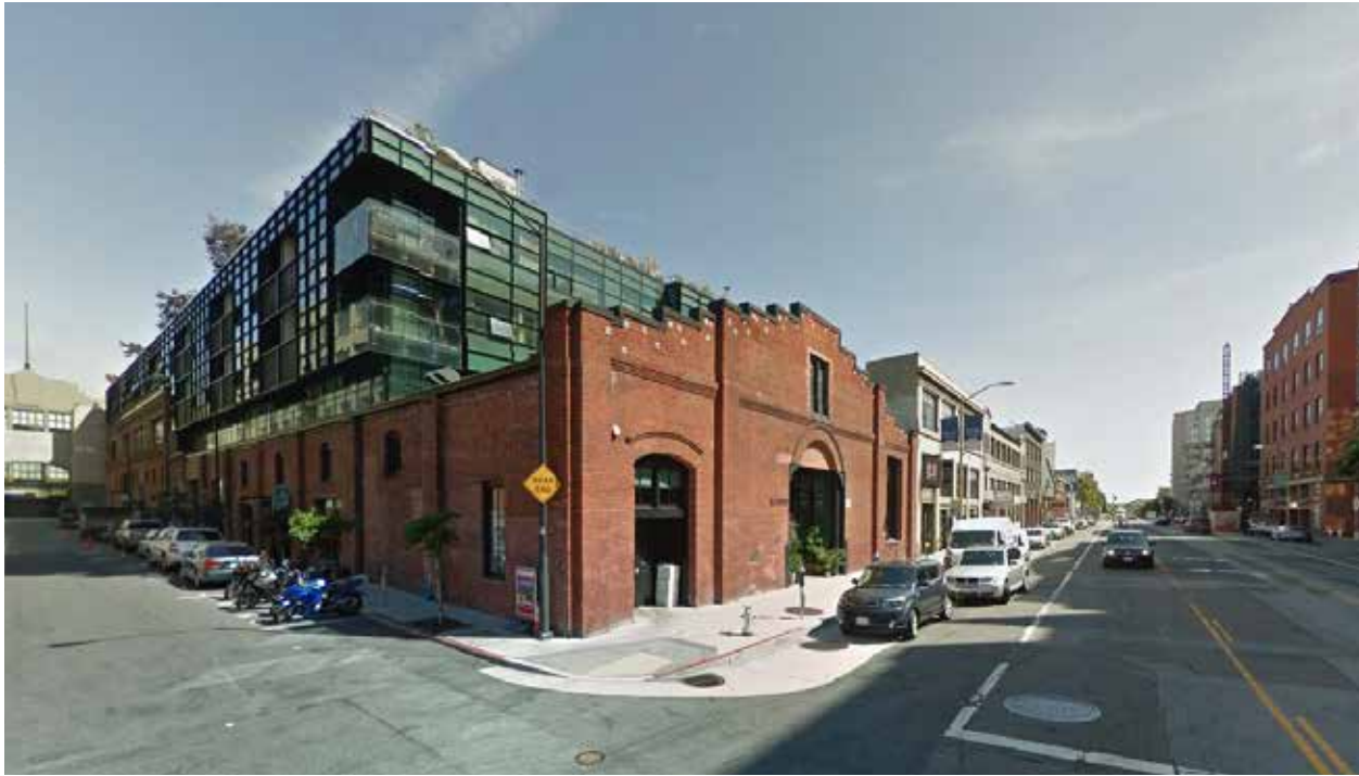
166–178 Townsend St (2016, After Construction)
