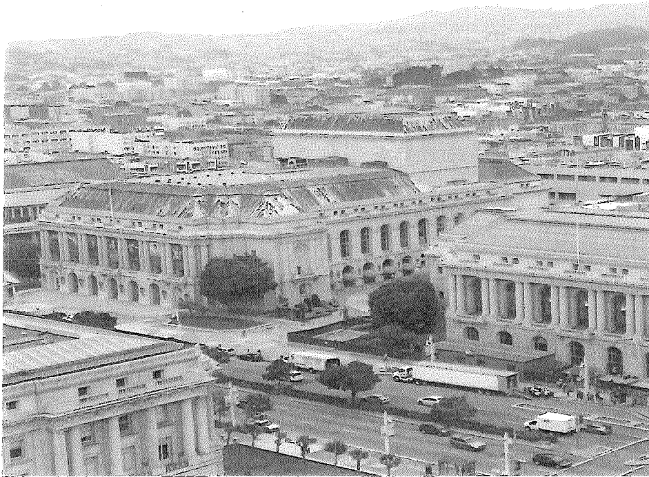
Opera House Roof: Solar PV System to be installed on flat roof; Mansard/sloped roof to be replaced.
