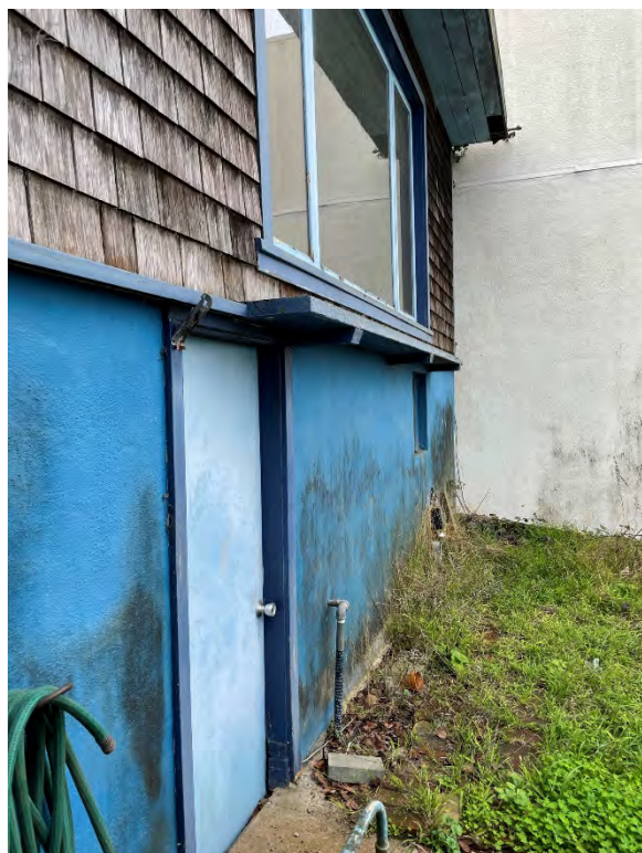
651 Duncan Street, façade and picture window, view west, 2020 Source: YA Studio
