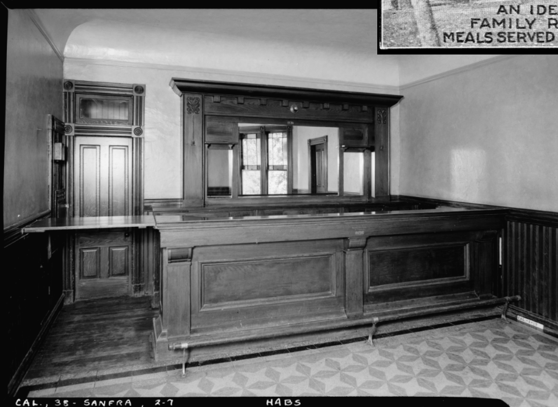
Trocadero Clubhouse, 1936 Bar Room
