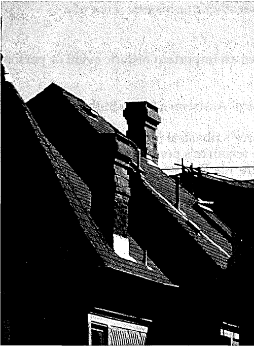
Figure 15. Detail of chimneys at south end of roof. (Photograph by Garavaglia Architecture, Inc., April 2015.)
