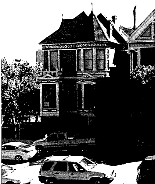
Figure 8. Overall view of west (Steiner Street) elevation. (Photograph by Garavaglia Architecture, Inc., April 2015.)
