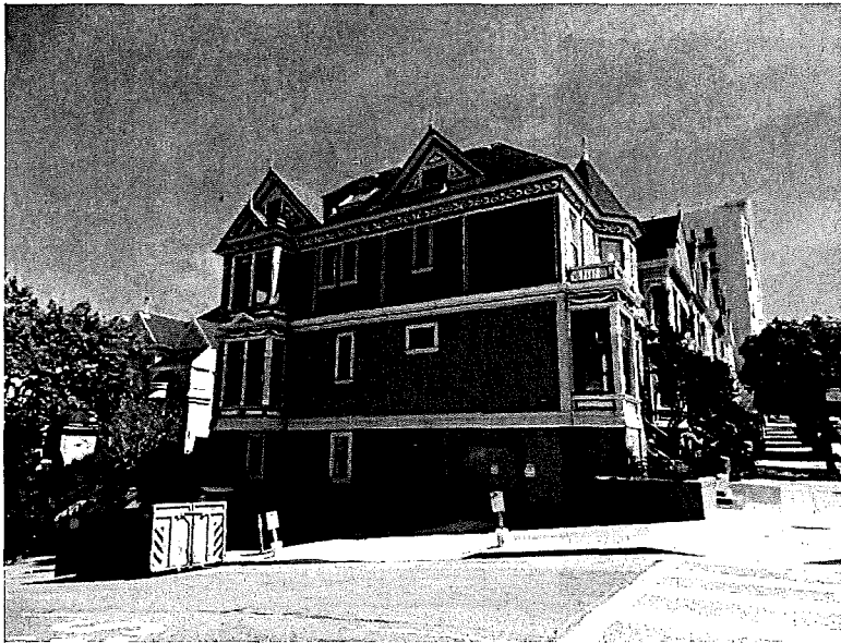
Figure 11. View of north (Grove Street) elevation, showing gabled dormers and fenestration. (Photograph by Garavaglia Architecture, Inc., May 2015.)
