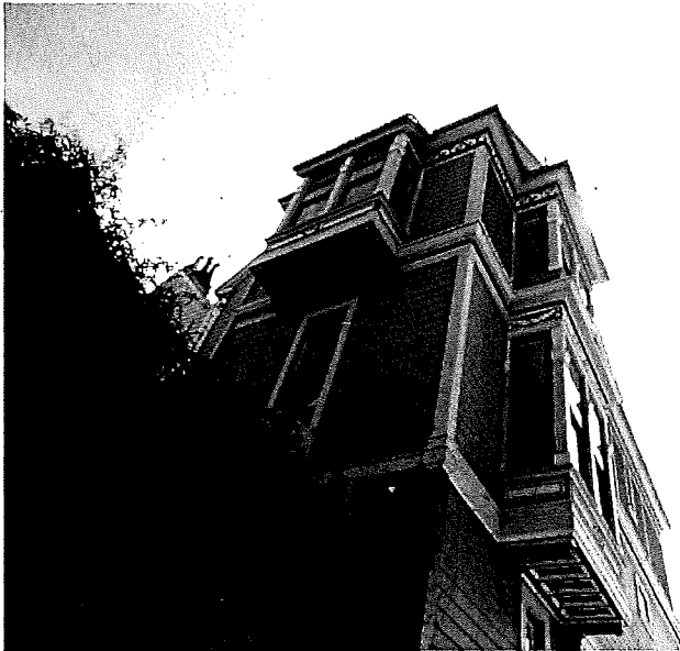
Figure 13. Partial view of the east (rear) elevation. (Photograph by Garavaglia Architecture, Inc., May 2015.)
