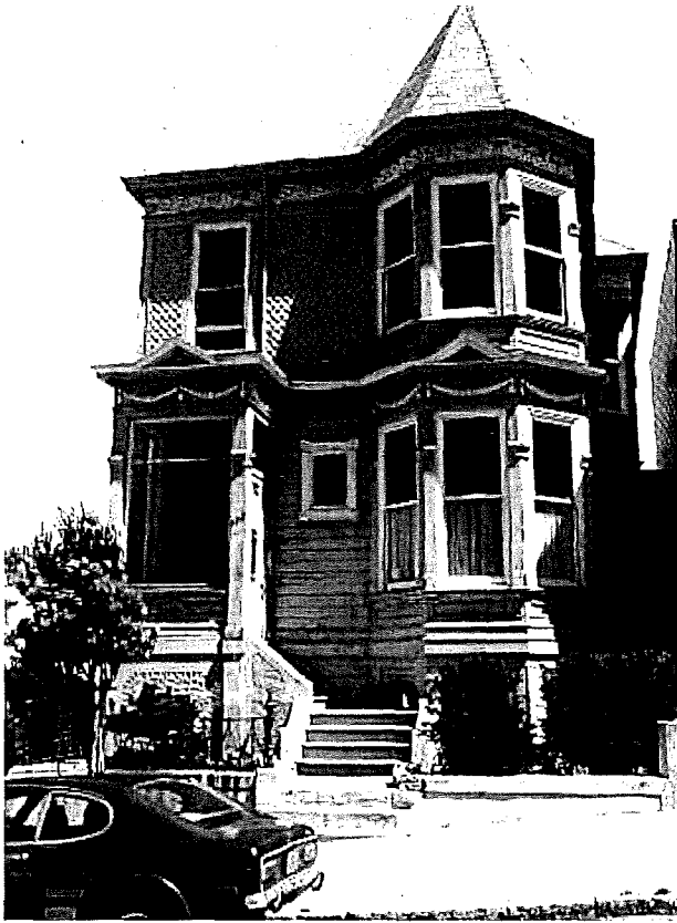
Figure 5. 722 Steiner Street, ca. 1976. In this photo, the portico has been closed in, and the exterior appears similar to how it looks today. The gate spanning the walkway to the south appears to be constructed of horizontal wood siding. (Photograph from San Francisco Planning Department, April 2015.)
