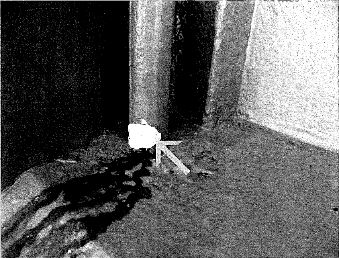
Corroded downspout
