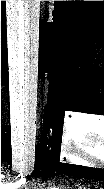
Figure 24. Rotted wood at entrance portico door. (Photograph provided by Côme Lague, April 2015.)
