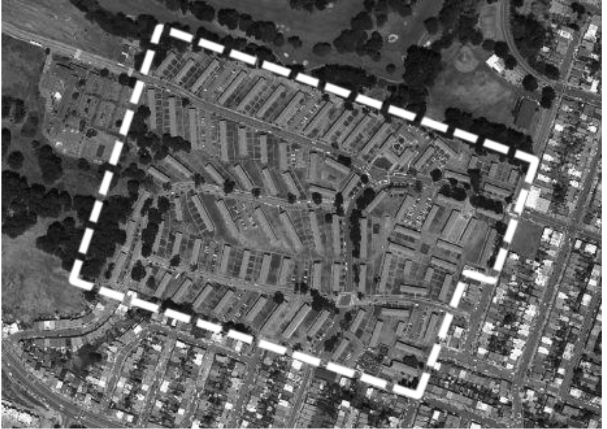
Existing aerial photo of 767 low-rise family townhouses at 16 units per acre
