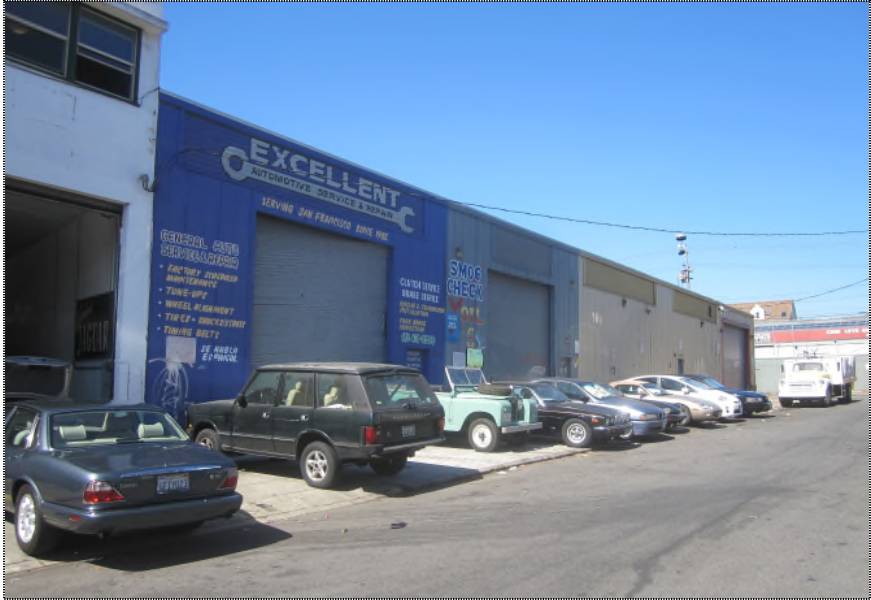
View of Subject from the Southeast
