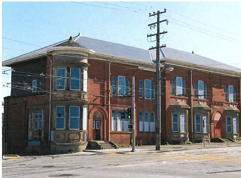
Figure 9. Geneva Car Bar and Power House
