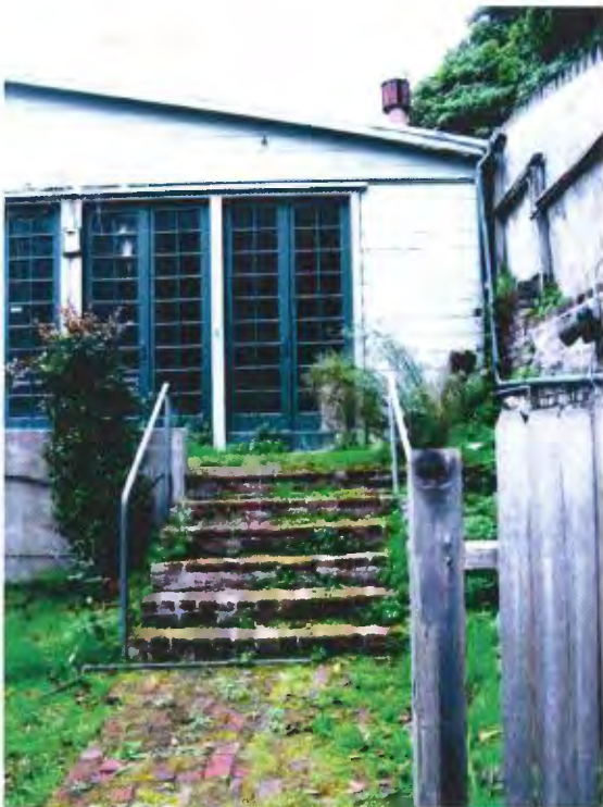
Figure 6. Detail of brick steps to be relocated. View north.
