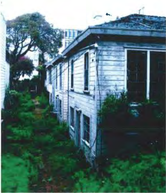
Figure 3. West facade of cottages. Note brick pathway. View north.
