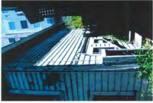
COTTAGE C South
