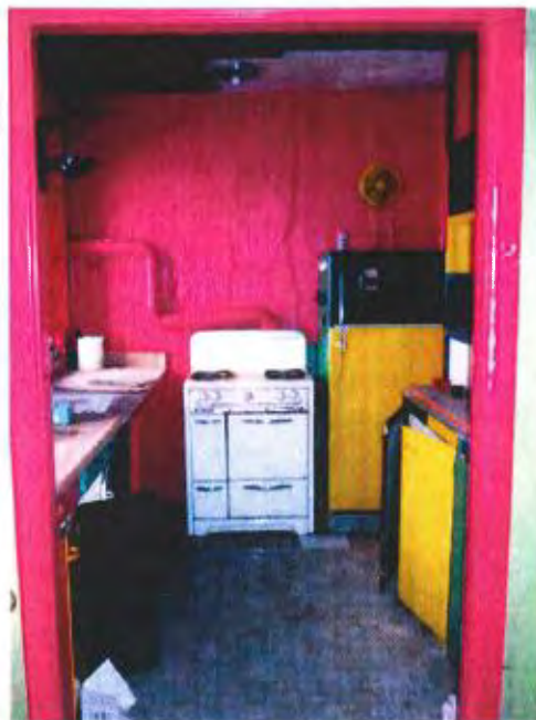
Figure 35: Existing kitchen, upper unit of Cottage D.
