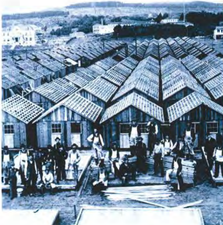
Figure 11. Richmond district refugee camp, 1906. Note roof construction consisting of rafters and purlins (San Francisco History Center, San Francisco Public Library).
