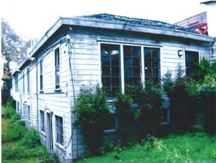
Figure 3: View of the primary (west) facades of the cottages and south façade of Cottage A. Note boxed eaves.
