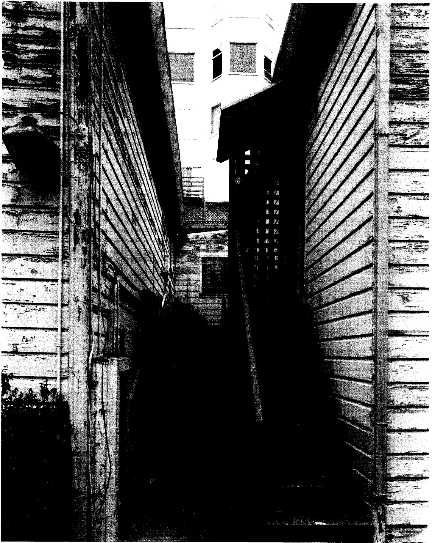
#6 VIEW OF COURT BETWEEN COTTAGES "B & C", LOOKING NORTHEAST
