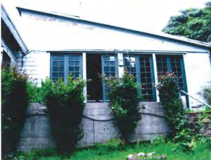
Figure 4. West facade of studio. View east.
