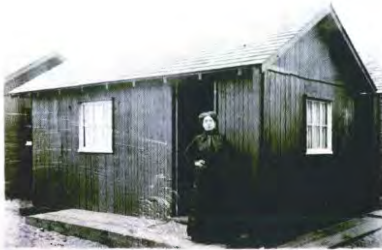
Figure 10. Earthquake shack, 1906. Note exposed rafter tails, wood shingles and round flue (San Francisco History Center, San Francisco Public Library).
