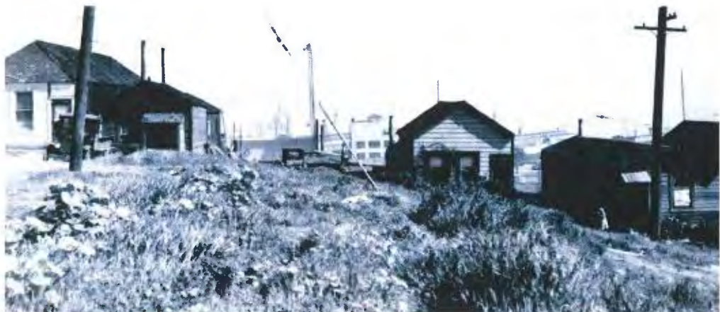
Figure 9. Row of shacks on First Street, 1934. Note shack at left with hipped roof clad in wood shingles (San Francisco History Center, San Francisco Public Library).
