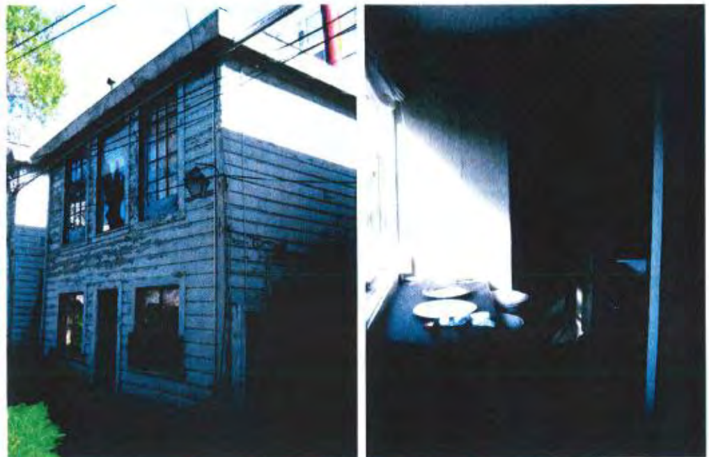
Figure 11 (right): interior Cottage C, lower unit kitchen, facing north.
