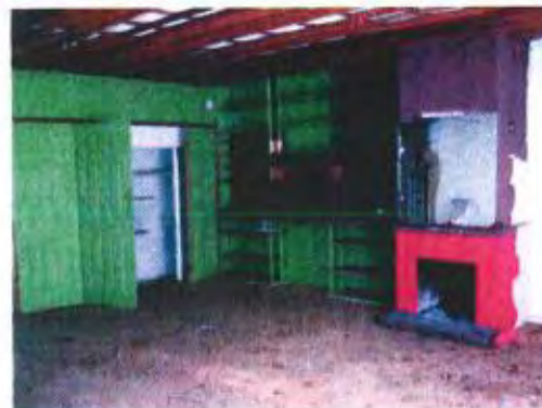
Figure 14 (bottom left): interior of Cottage D, main room, facing southeast.
