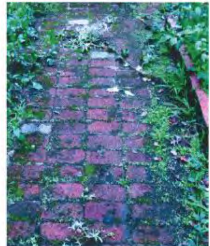
Figure 4: Walkway showing “stacked” coursing and raised brick planter
