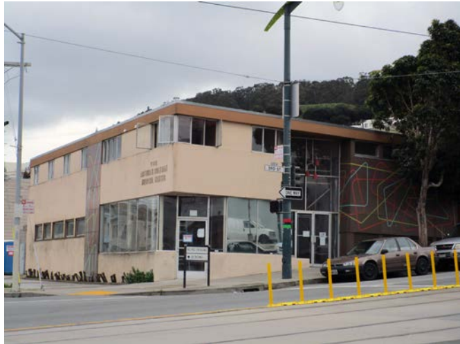
The historic Arthur H. Coleman Medical Center at 6301 Third Street, view southeast.
