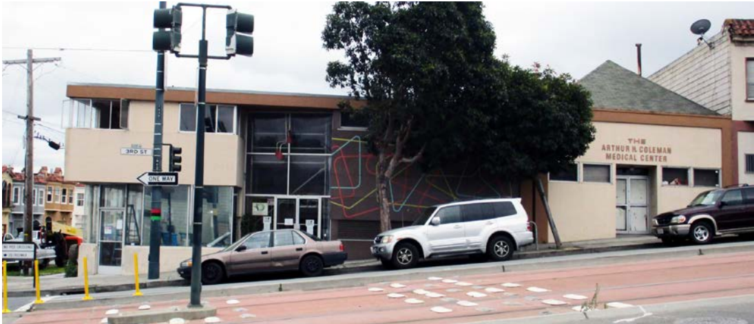
Primary (west) elevation, view east.
