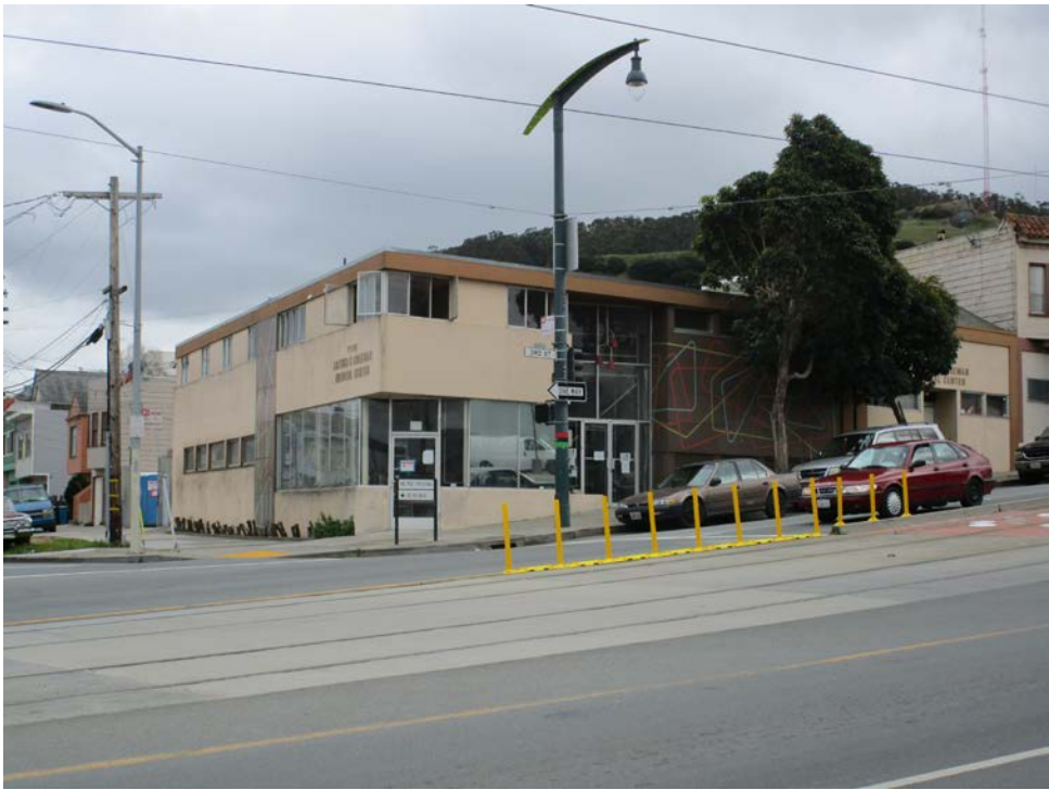
Primary (north and west) elevations, view southeast.
