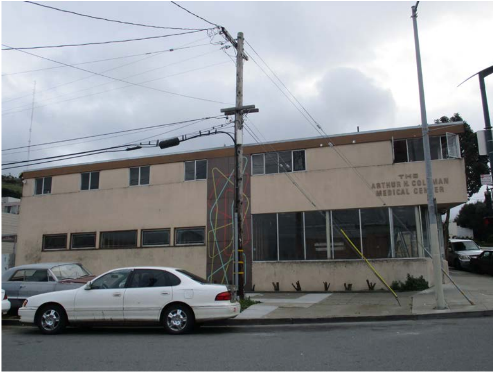
North (Ingerson Avenue) elevation, view south.
