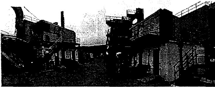
Electrical Power Room (bottom) and Control Room (top), northwest facing elevations (left) and southwest facing elevations (right)
