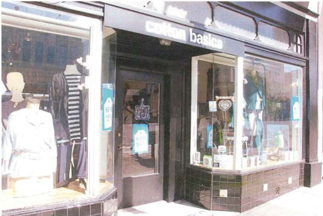
Figure 5: An example of an intact storefront along the 24 th Street commercial corridor historic district, view southeast, 2015. Note the decorative square glazed tile at the bulkhead, seamless butt glazed storefront glass, and elaborate transom with translucent decorative glass.
