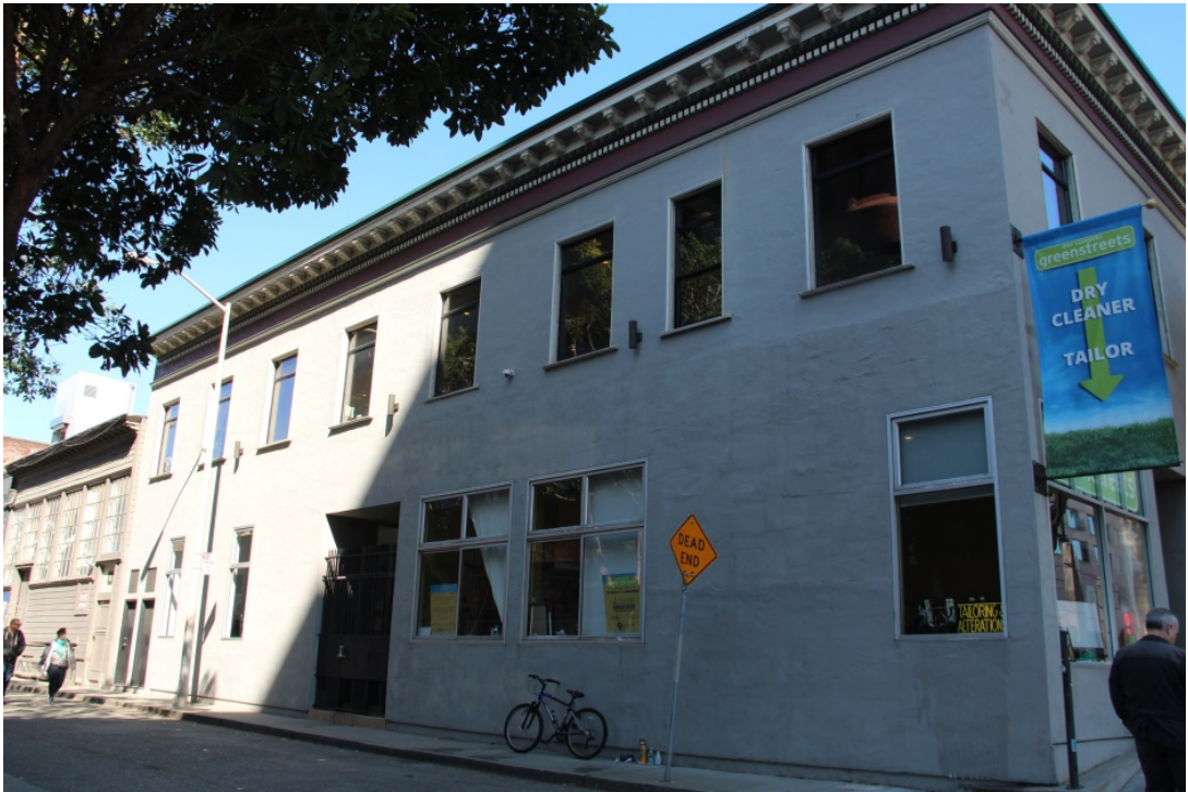
Secondary elevation (Lust Street), view north.
