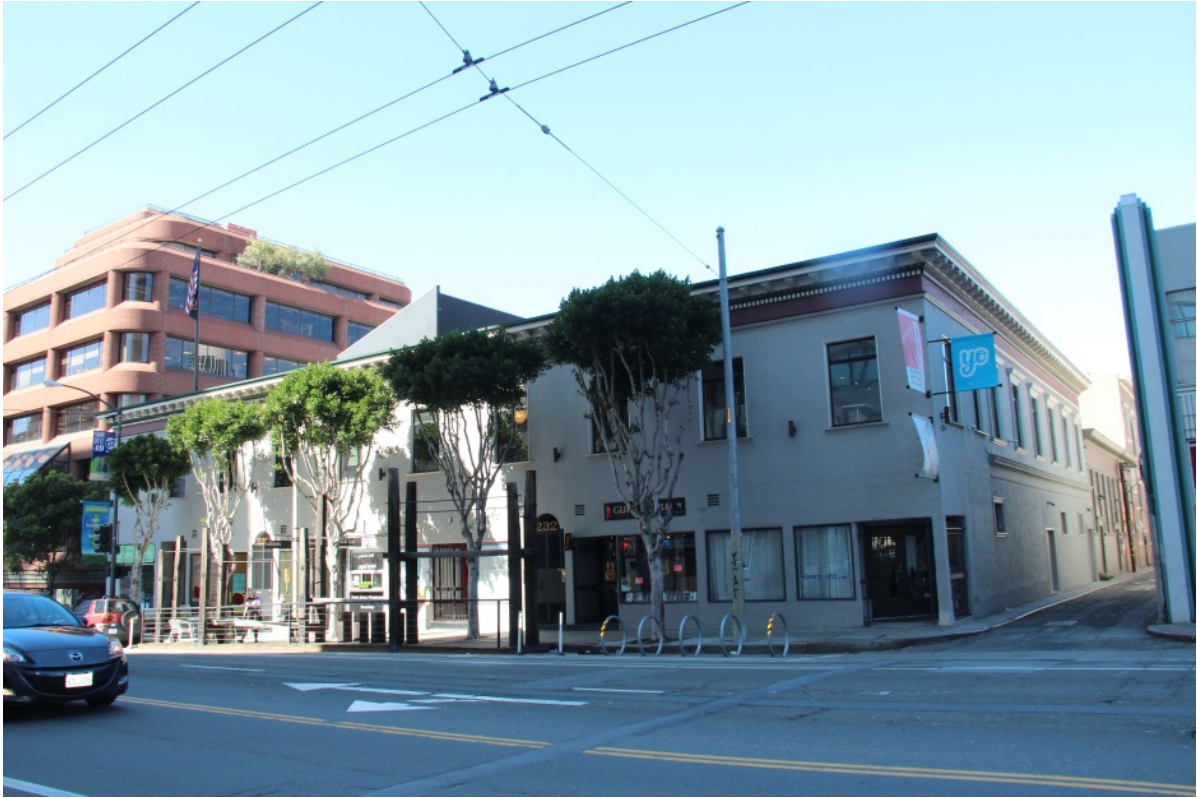
Primary elevation, view west.
