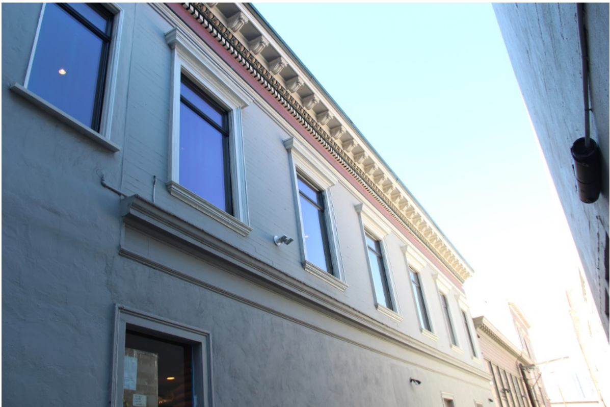
Secondary (Clyde Street) elevation, view west.
