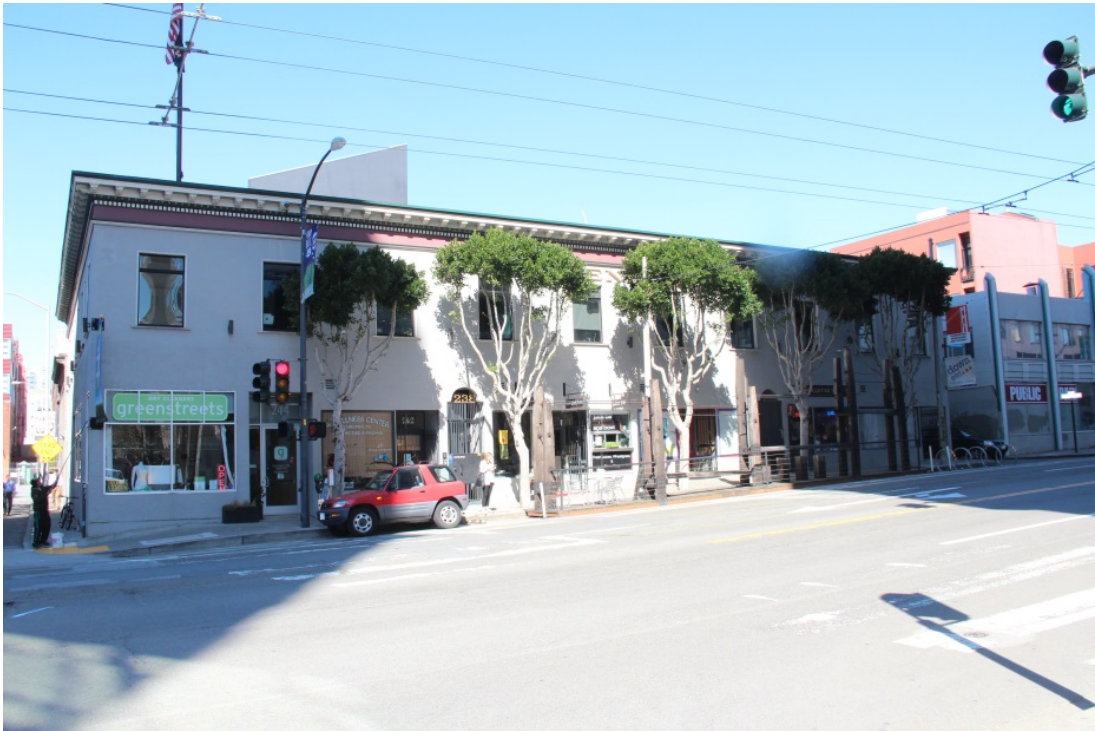
Primary elevation, view northwest.
