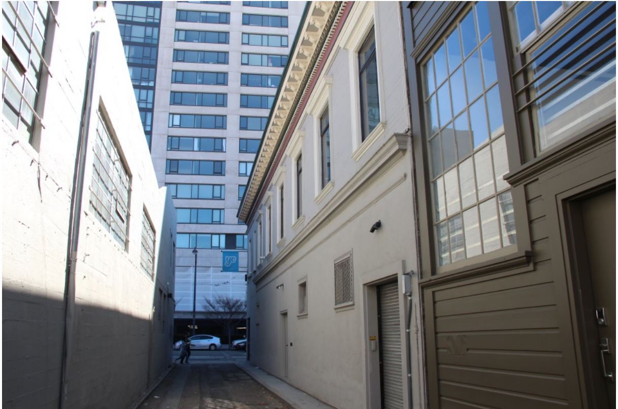
Clyde Street, view southeast. 228-248 Townsend Street is to the right.
