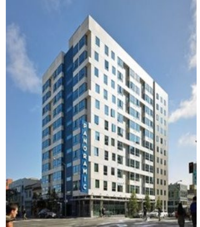
Newly acquired site for family and adult permanent supportive housing at The Margot (1321 Mission Street).
