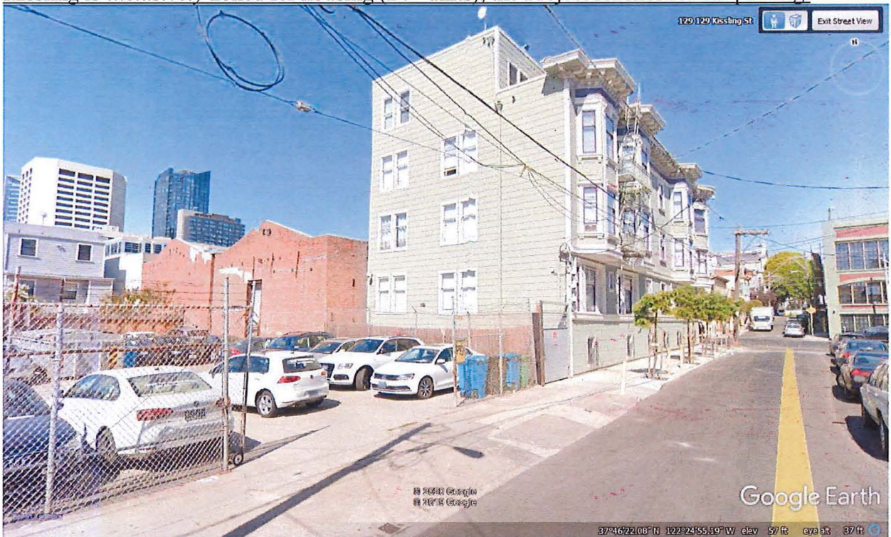
Kissling Street is in a Historic District and is zoned residential only enclave (RED), the proposal to intensify the non-conforming use for more cars on “stackers” and modern metal screens more than thirty (30’) feet tall is not compatible and lacks CEQA review.
