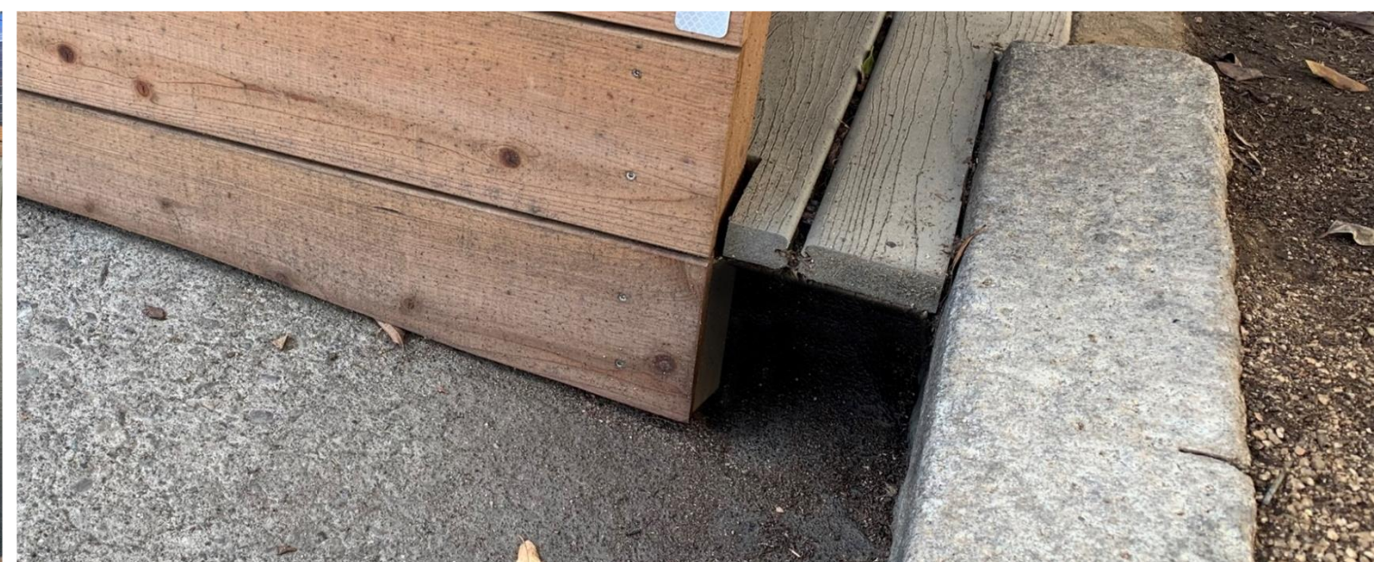
6 x 6 Inches Clear along Gutter
