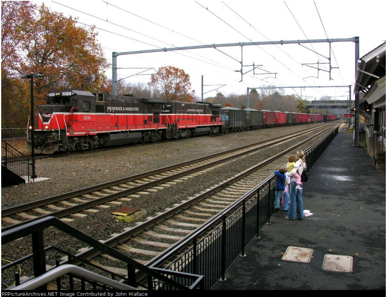
1 Figure B: Photograph of Providence and Worcester freight railroad operating on shared 2 tracks with electrified 25 kV overhead contact system overhead on the Northeast Corridor
