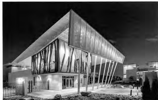
Figure 13: A Long Term Care Facility in LZ 3 with well-shielded lighting – no uplight. (Image courtesy of David Roederer)
