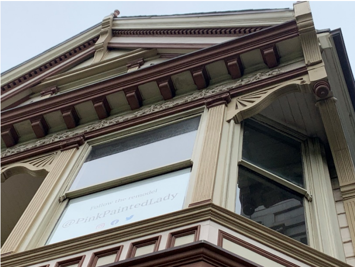
Bay Window detail
