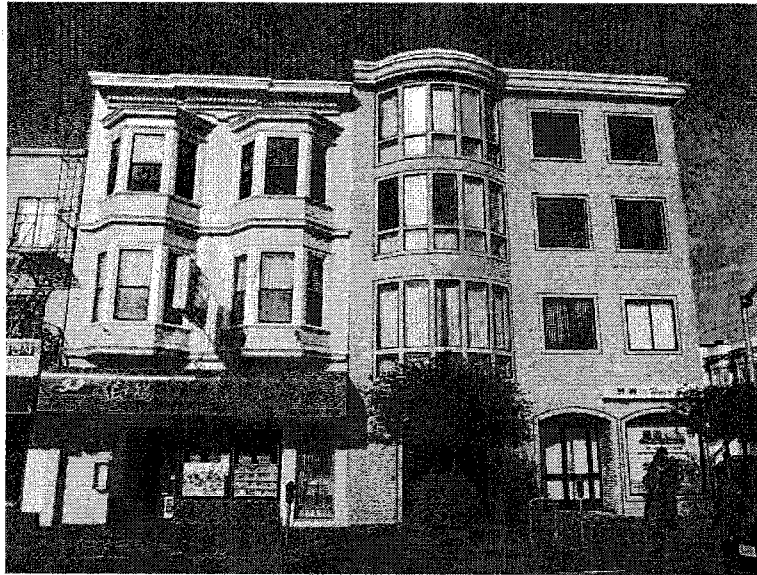
Figure 1- Located on Geary Boulevard and 4 th Avenue, these two buildings speak to the benefit of proposed Ordinance in enhancing the street frontage of buildings. The building on the right is a newer four story building with an inactive and lower ceiling ground floor. The building on the left, almost equally as tall, only includes three floors but more active and higher ceiling ground floor. An additional maximum five foot for the building on the right, could have improved the ground floor while maintaining the four stories.
