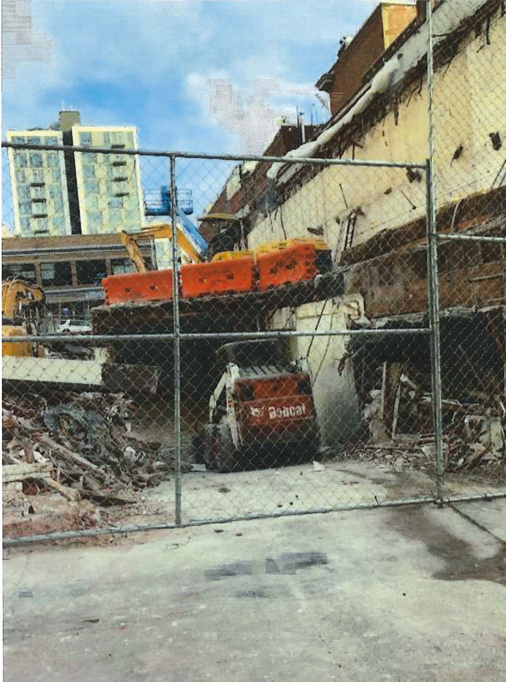
Figure 7 1433 Bush Street Demolition using small tools
