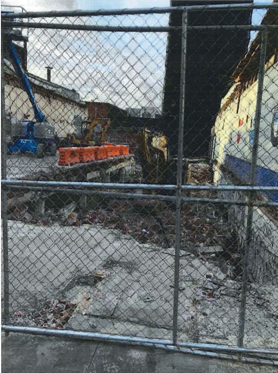
Figure 6 1433 Bush Street Demolition, Excavation and shoring 6,000 CY
