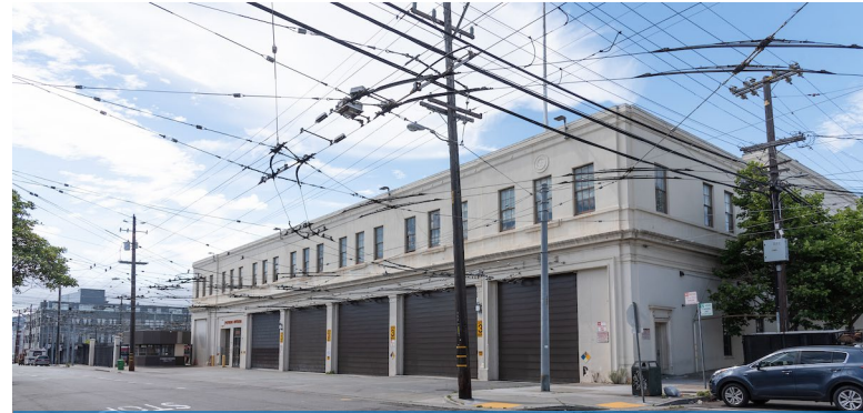
Seismic Upgrades & Building Replacement
